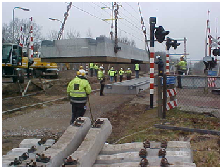
Figure 22 - Example installation of pre-cast slab track level crossing
