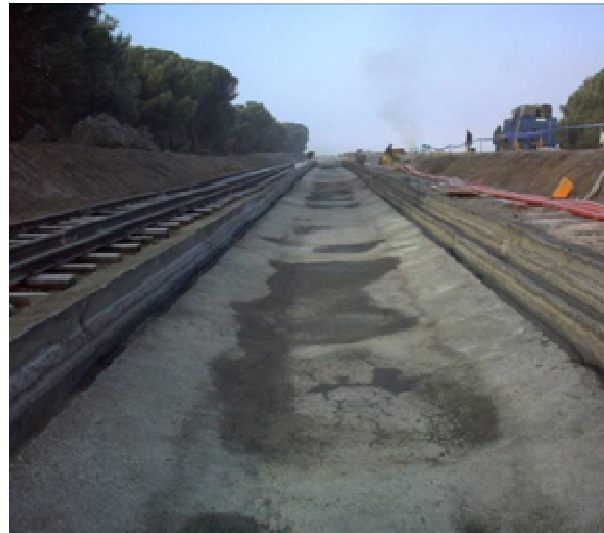
Figure 23 - Example installation of cast in-situ track slab in Spain
