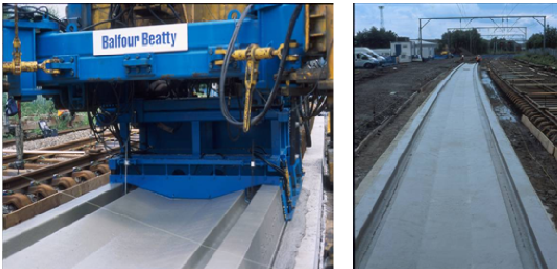
Figure 21 - Slip formed slab at Crewe
