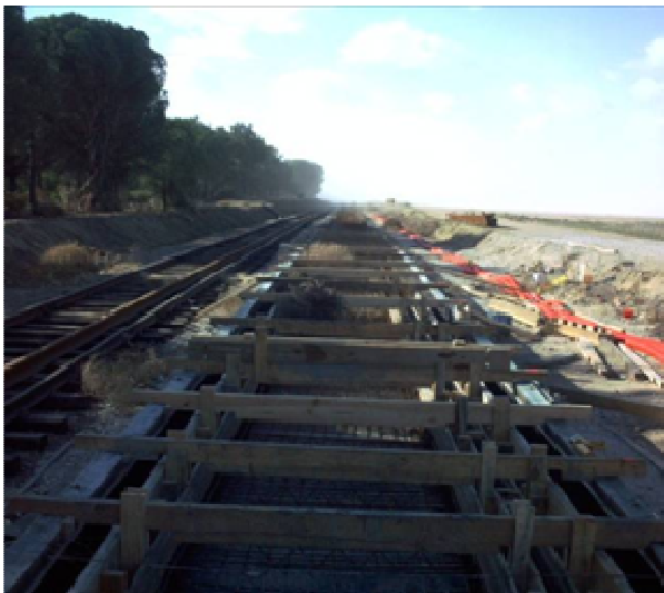
Figure 23 - Example installation of cast in-situ track slab in Spain
