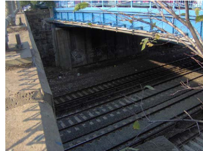
Parcel B6600, between Mosholu Parkway and parking deck
