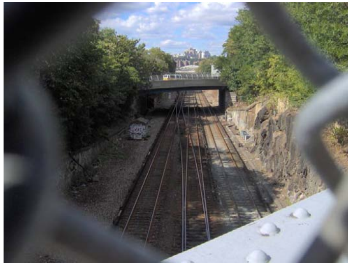
Parcel B6701, looking north from Walton Avenue towards Gerard Avenue
