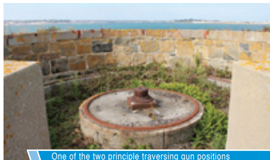
One of the two principle traversing gun positions on the top of Brehon Tower (H Glencross)
