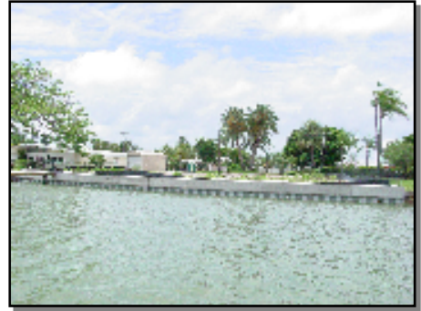
Seawall along an altered shoreline
