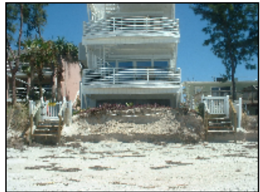
Dunes helped protect this home during the 2004 hurricane season
