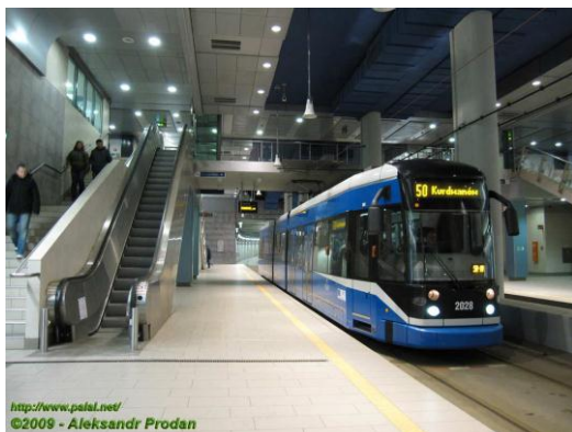
Figure 5.7 A mezzanine at a tram station in Krakow, Poland (Prodan, 2009).
