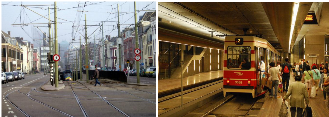
Figure 4.1 West tunnel entrance from street running tracks (Archined, 2004) and interior of station at Haag tramway tunnel (Flickr.com, 2009).
