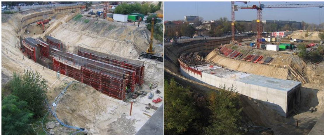
Figure 4.3 Construction of a cut-and-cover tunnel in Krakow, Poland (Skyscrapercity Forums, 2007).
