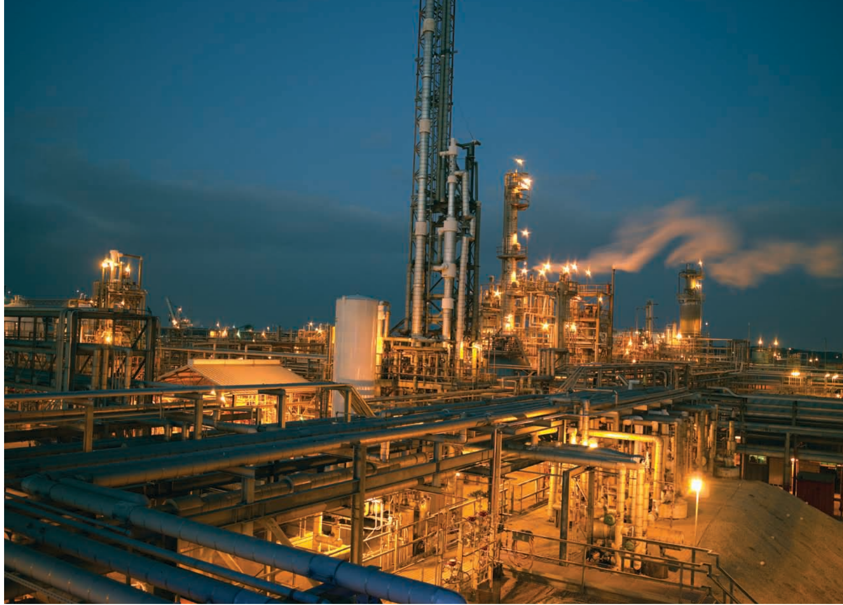
MEMC's Pasadena plant, 2007.
