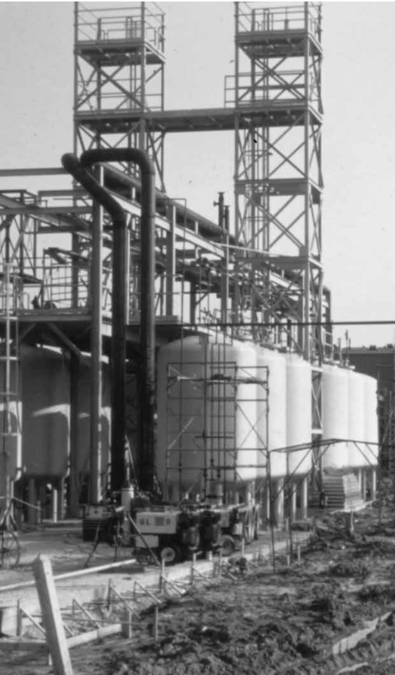
Distillation columns at the St. Peters expansion, 1970.
