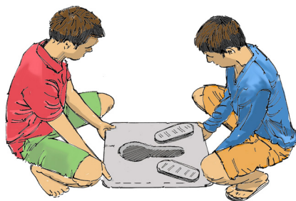
Figure 18. Lifting a sanplat
