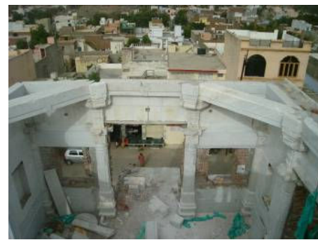
Figure 43.1 & 43.2 -Process of fixing of the roof slabs (Source: www.himalayanacademy.com )
