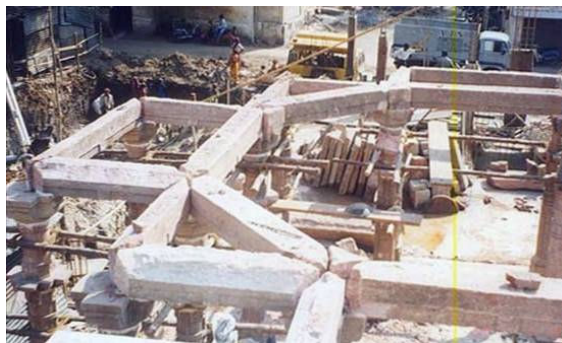
Figure 43.1 & 43.2 -Process of fixing of the roof slabs (Source: www.himalayanacademy.com )
