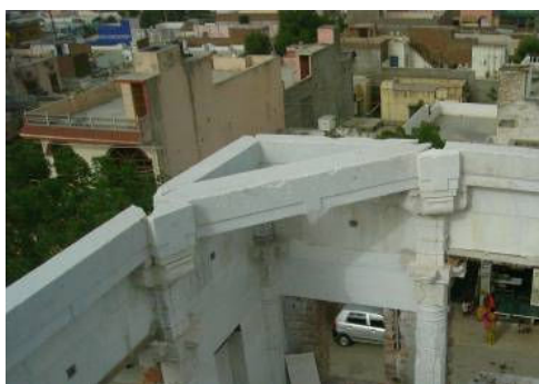
Figure 44-Arrangement of the beams and roof slabs for the mandapa ceiling.(Source: www.sompura.com & author's collection)
