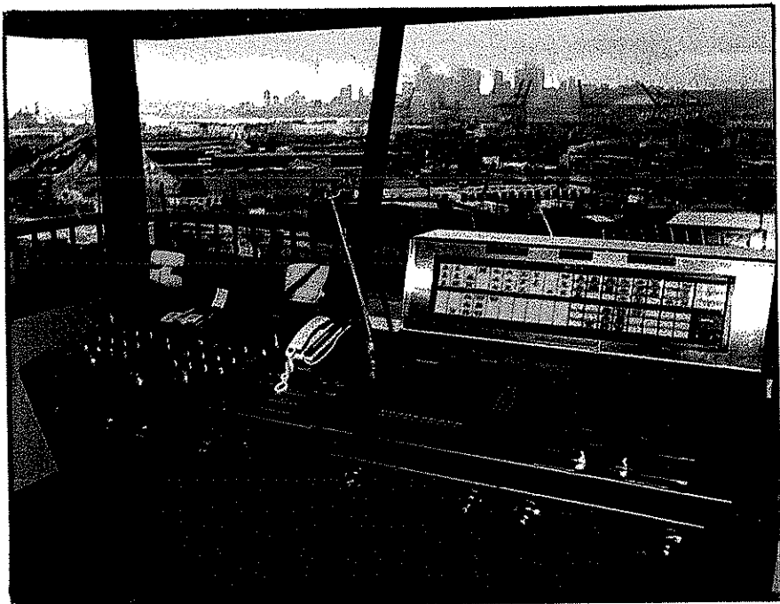
Bridge Operator Control Console
