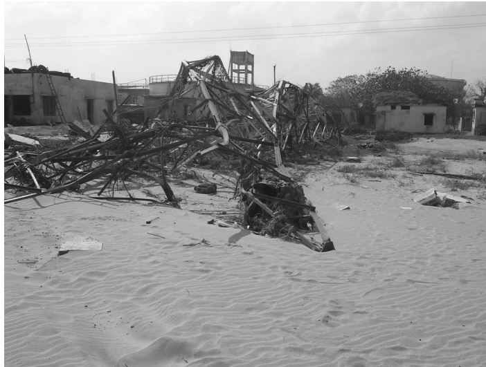
Figure 19. Damaged communication tower on Ariyanattu Street (photo: A. Sheth).
