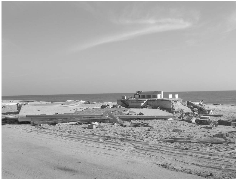
Figure 16. Some homes at Melamanakudi were within 6 m of the shoreline. This photo shows a fallen RC roof slab (photo: A. Sheth).
