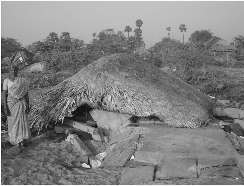
Figure 30. Fishermen's huts of adobe and mud plaster walls were razed at Prakasham (photo: A. Jaiswal).
