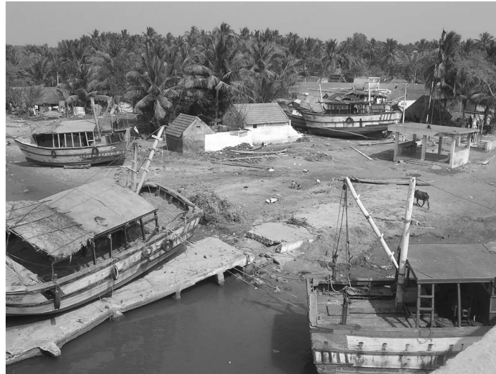
Figure 24. At Singarathop, the bridge from which this photo was taken is much higher than the town and served as a refuge (photo: A. Sheth).
