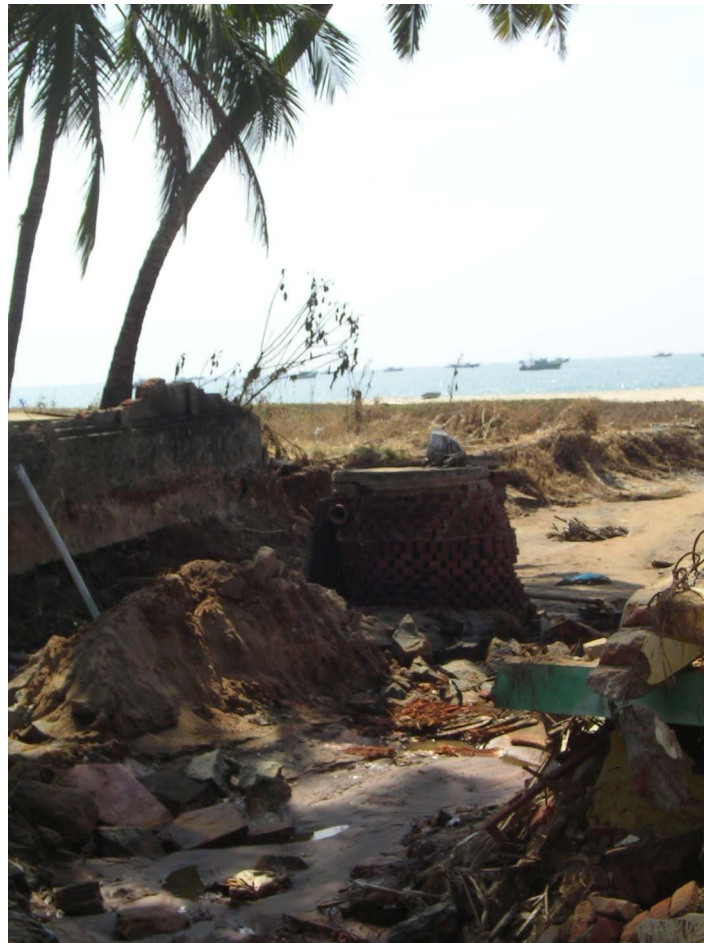
Figure 11. The tsunami carved new waterways—a soak pit was exposed by tsunami waves in Kolachel (photo: A. Sheth).
