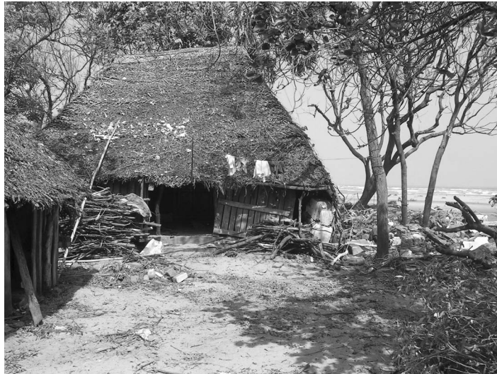
Figure 18. Houses in Seruthur, the village neighboring Velankanni, were not significantly affected, due to a higher plinth (photo: A. Sheth).
