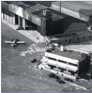
Terminal building in 1947 with the 'crows nest' shed forming the control tower on top of the still-camouflaged hangar
