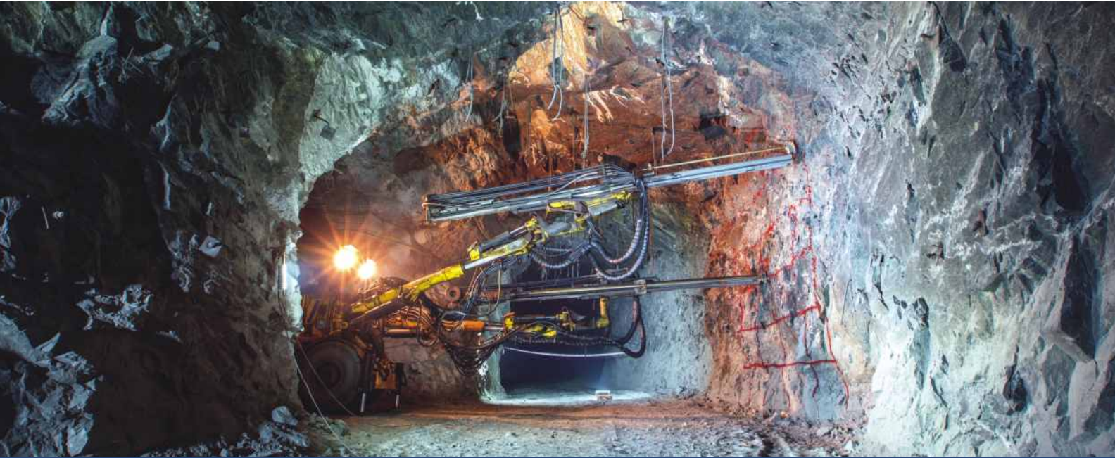
Double Drill Jumbo at work in Sindesar Khurd Mine
