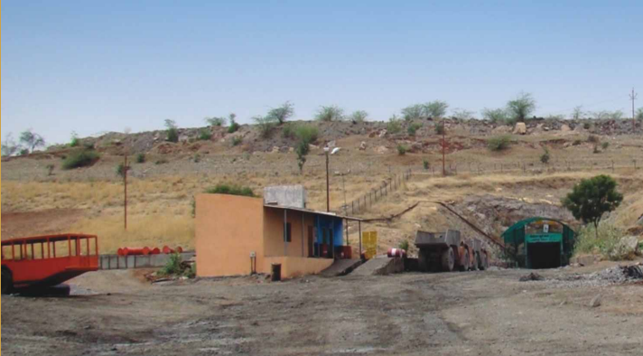
Sindesar Khurd Mine main entrance
