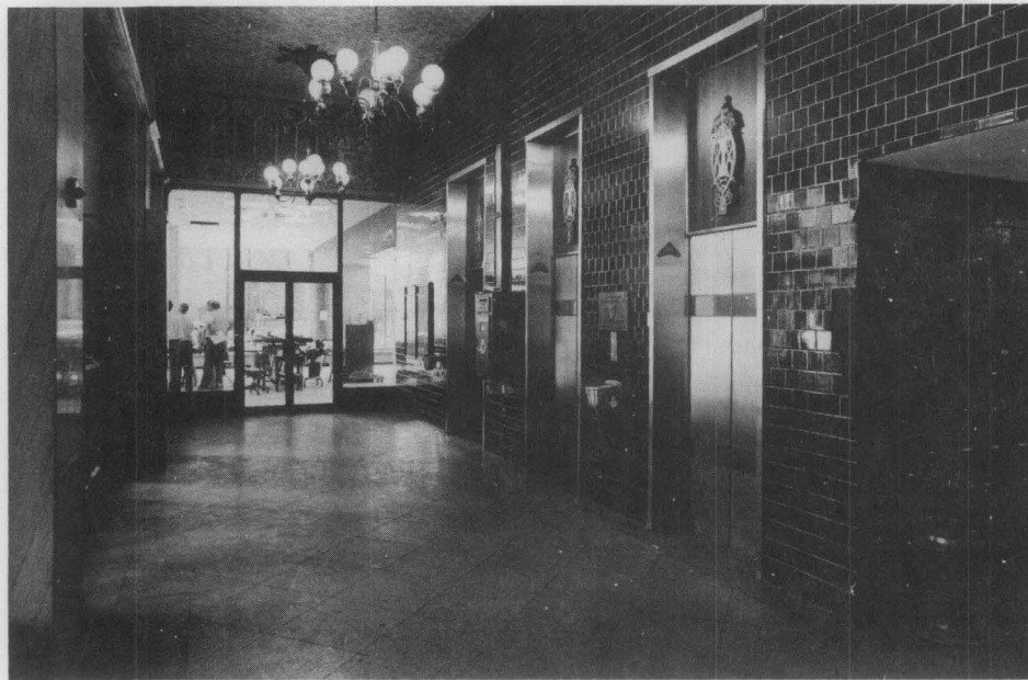
Figure 3. First floor elevator lobby, c. 1962. Modifications included reduction in number of elevators and addition of masonry enclosure around open elevators and main building stair. Photo: Cannon.
