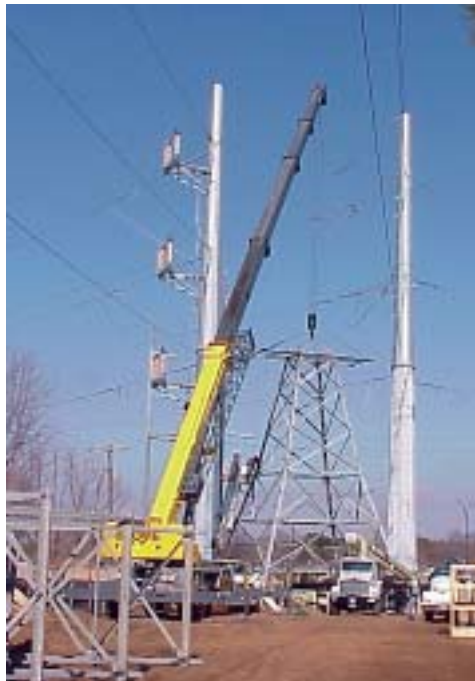
A crane is used to rebuild a tower behind a residential development along the Everman to Handley route.
