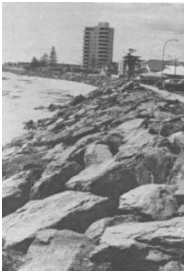
Rip-rap Wall - North Glenelg
