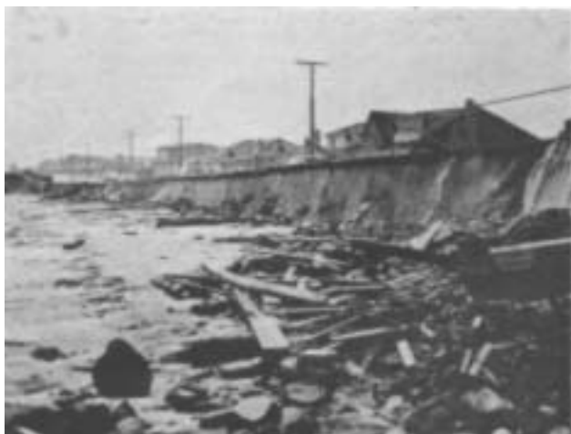
Storm Damage - Glenelg, 1964
