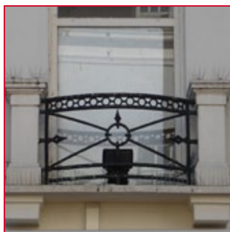
Convex iron frontal across first floor window.
