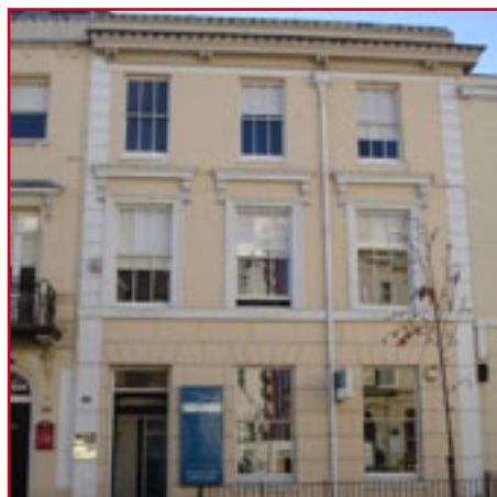
Windows in an Italian style with deep bracket cornice and banded pilasters.
