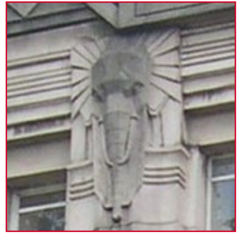
Upper storey detail on 4 - 6 Queen Street.
