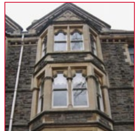
The strong shape of the window heads varies at each floor level – 9 & 10 Park Place
