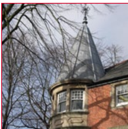
A lead covered turret turns the corner on Park Place.
