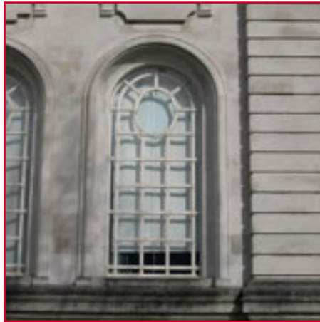
Metal windows create elegant building details.
