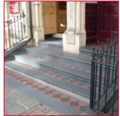
A modern restoration of tiled steps to a paired porch area.
