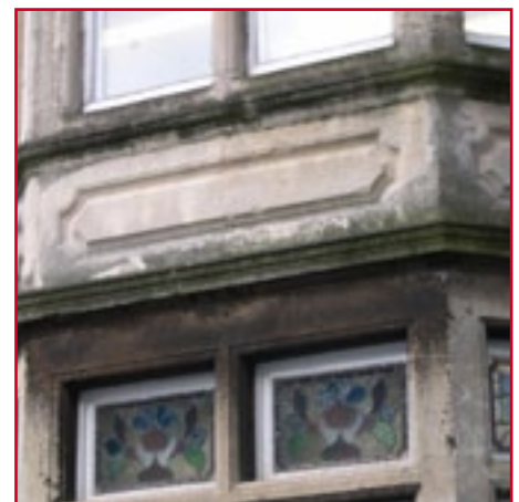
Leaded lights within a stone bay.
