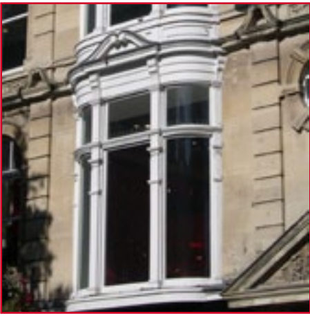
Victorian window detailing at the Andrews Building.
