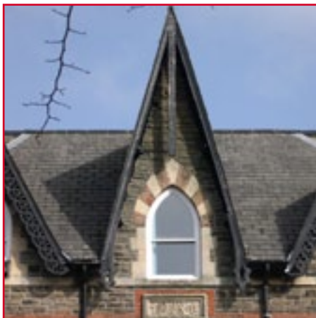
Brick and stone is used to decorative effect around this gabled dormer on Park Place
