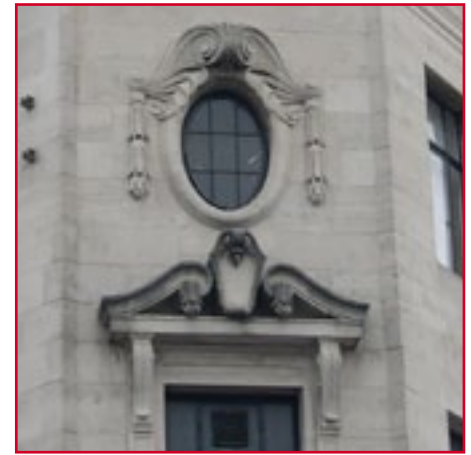
Carved stone around openings, 2 Queen St.
