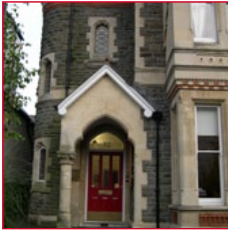
A bath stone porch on Park Place with pennant stone behind.
