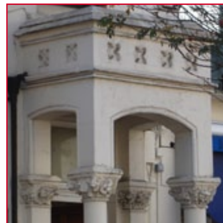
Open porch with quatrefoil banding and columns with annulets and foliage capitals.
