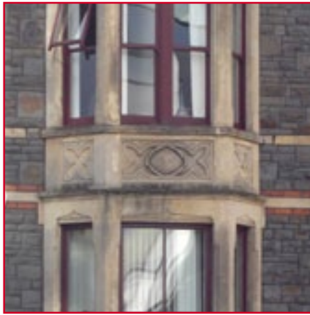
Bathstone bays with decorative panels.
