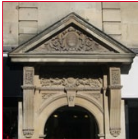
Carved stone over door-way, the Andrews Buildings.
