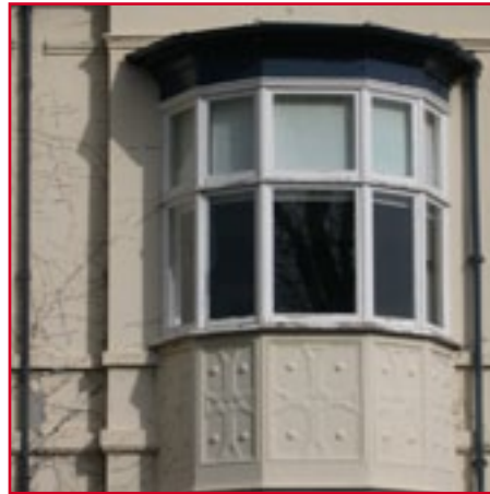
A mid 19th C stuccoed bay with decorative finish.
