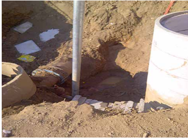
Fig. A4.1. Water pipeline thrust block supported by a sewer manhole
