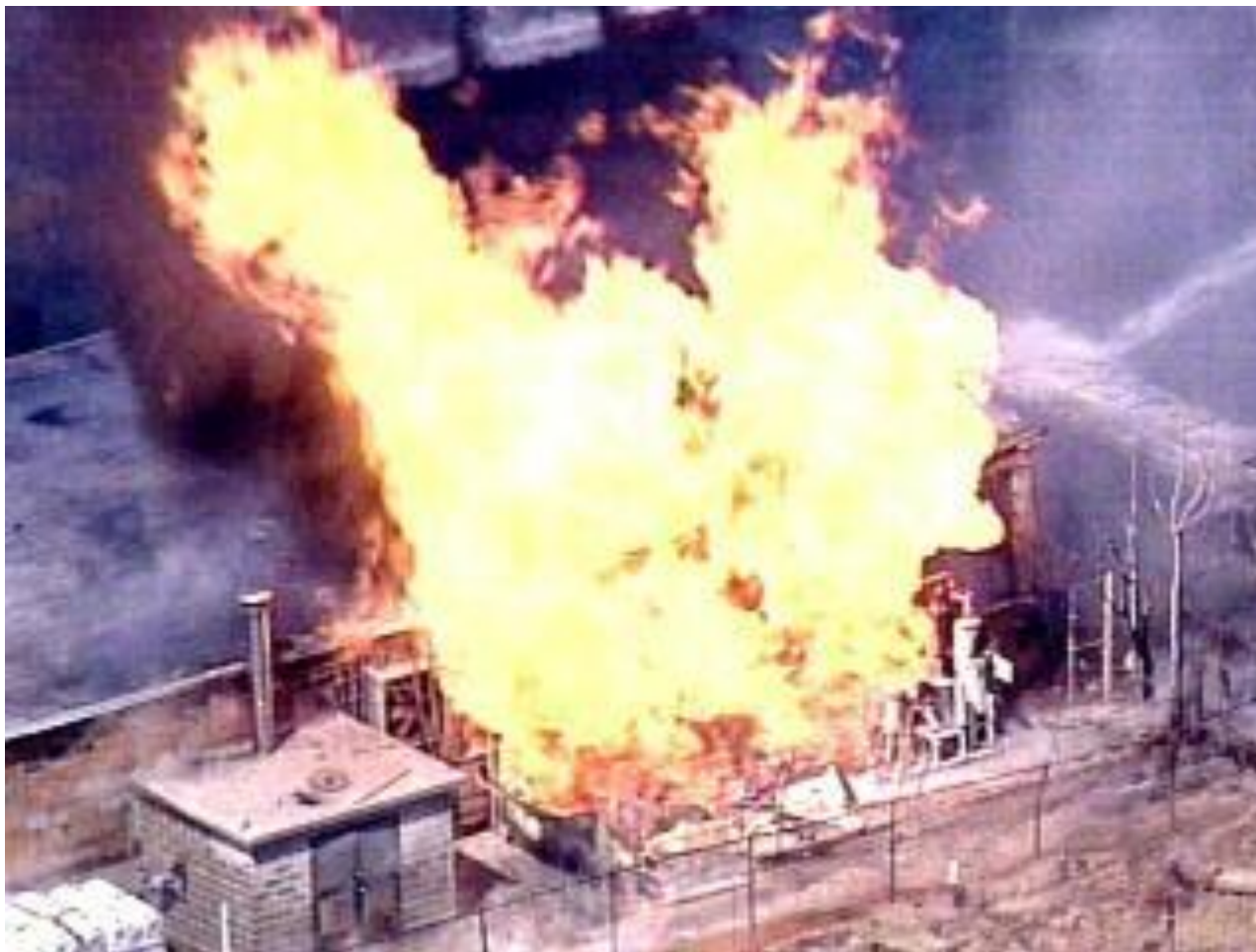
Inherited Unsafe CNG Fueling Station at LaGuardia Depot
