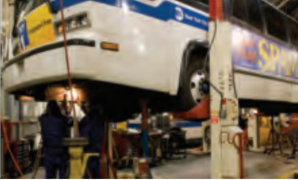
New portable lifts are improving maintenance at the Manhattanville and other depots
