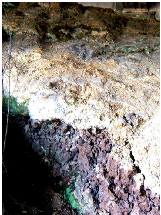
Fig.3: Part of the exposure of Mt Hobson lava flow and weathered soil overlain by lighter coloured tuff (inferred to be from Three Kings Volcano) located beneath the Market Rd bridge over the Southern Motorway, 2009.
