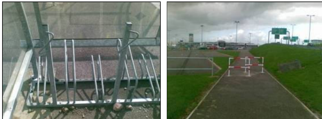
Figure 4-5 Existing Cycle Parking Stand Figure 4-6 Obstruction on existing cycle lane
