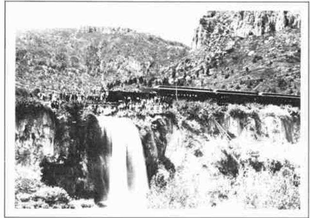
The Chicago, Burlington and Quincy Railroad (above far left and above) traversed Spearfish Canyon in the days before highway travel. It was a popular and spectacular trip for the Black Hills tourist. Fishermen rode the railroad to their favorite fishing spots in the canyon. It also made stops in the canyon along the creek to accommodate the traveling fisherman, first leaving him off at a likely spot and then picking him up on the return run, 1910.
