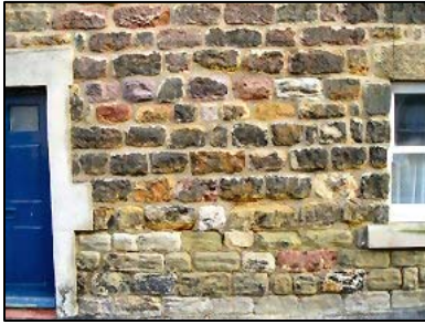
Typical sandstone walling - Northumberland Street
