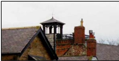
Roof details - Northumberland Street
