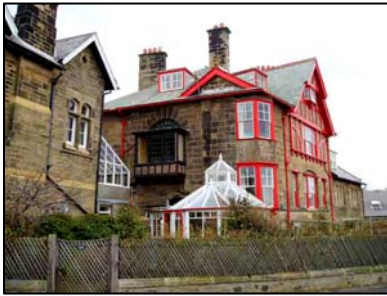
Un-neighbourly paintwork spoils a fine building and conservatory - Marine Terrace
