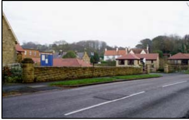
Loose grouping of buildings - Friary Gardens
