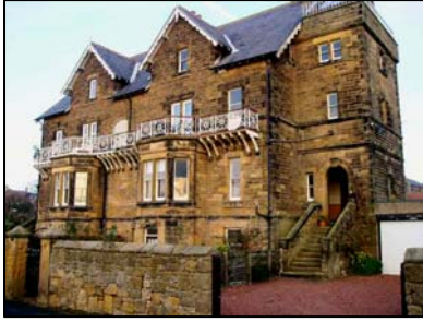
Bargeboards and balconies - Riverside Road
