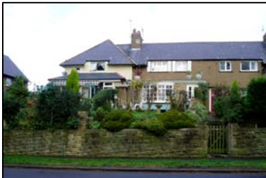
Replacement windows and other incremental changes - B1338
