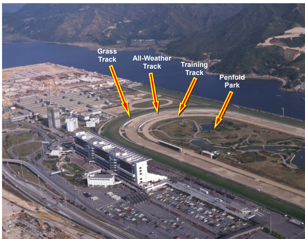
Fig. 4.1: Aerial view of STRC, 1981
