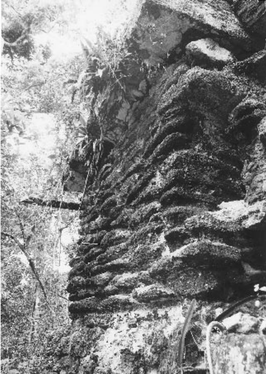
Fig. 28 Wall exterior of Structure 34, El Mirador. Note the evenly shaped stone blocks and cornice stones.
