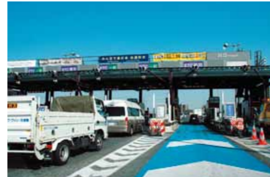
ETC for non-stop toll collection has been installed at almost all expressway toll gates in Japan, contributing toward mitigating toll-booth congestion.
