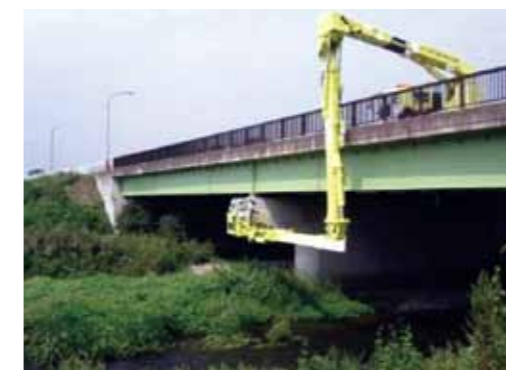
Bridge inspection example
