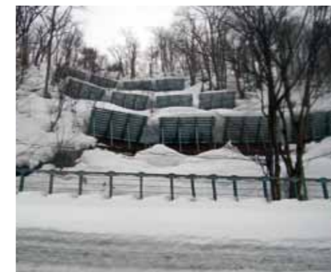
Snow shed that provides avalanche protection
