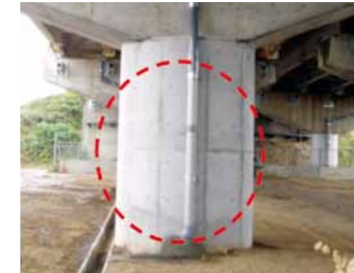
Bridge pier seismically reinforced by concrete jacketing
