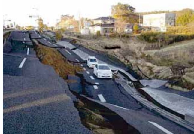
Massive earthquake and the following giant tsunami on the 11th of March 2011 caused enormous damages to the roads (National Highway 6, Hirono-machi, Fukushima Prefecture) (Photo: Tohoku Regional Development Bureau)
