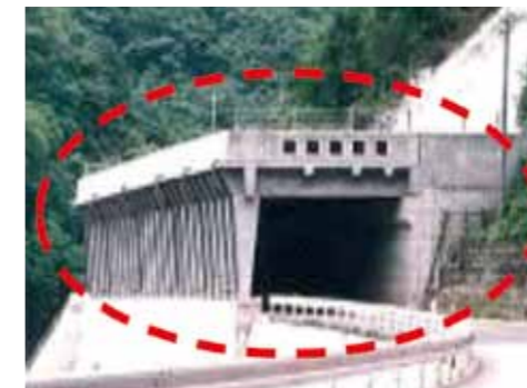
Road with rockfall shelter
