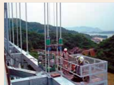
Non-destructive inspection of hangers
