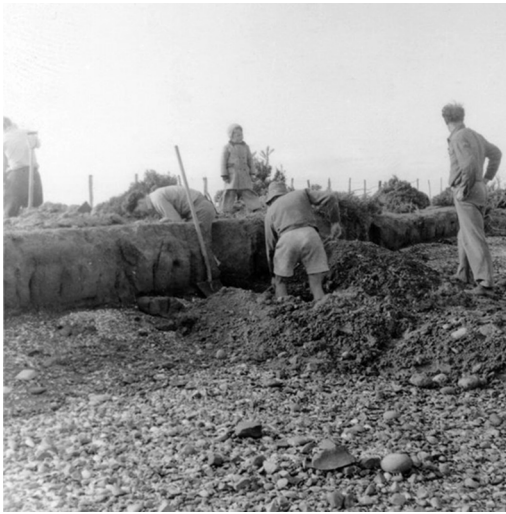
Figure 22. Excavation of one of the lagoon trenches (photo, Canterbury Museum)
