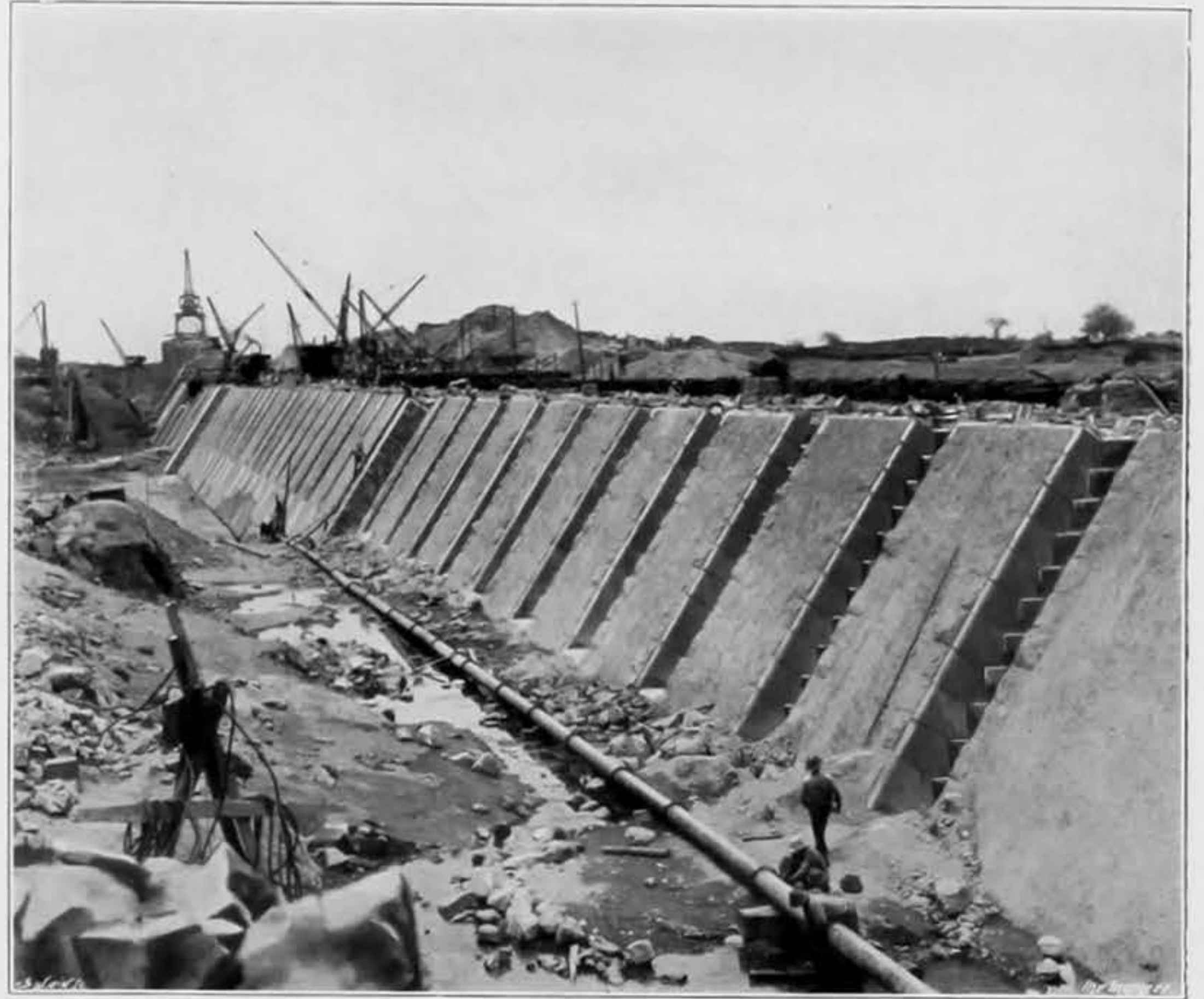
FIG. VI.—DOWN-STREAM FACE OF EASTERN PORTION OF DAM—JULY 1, 1924
