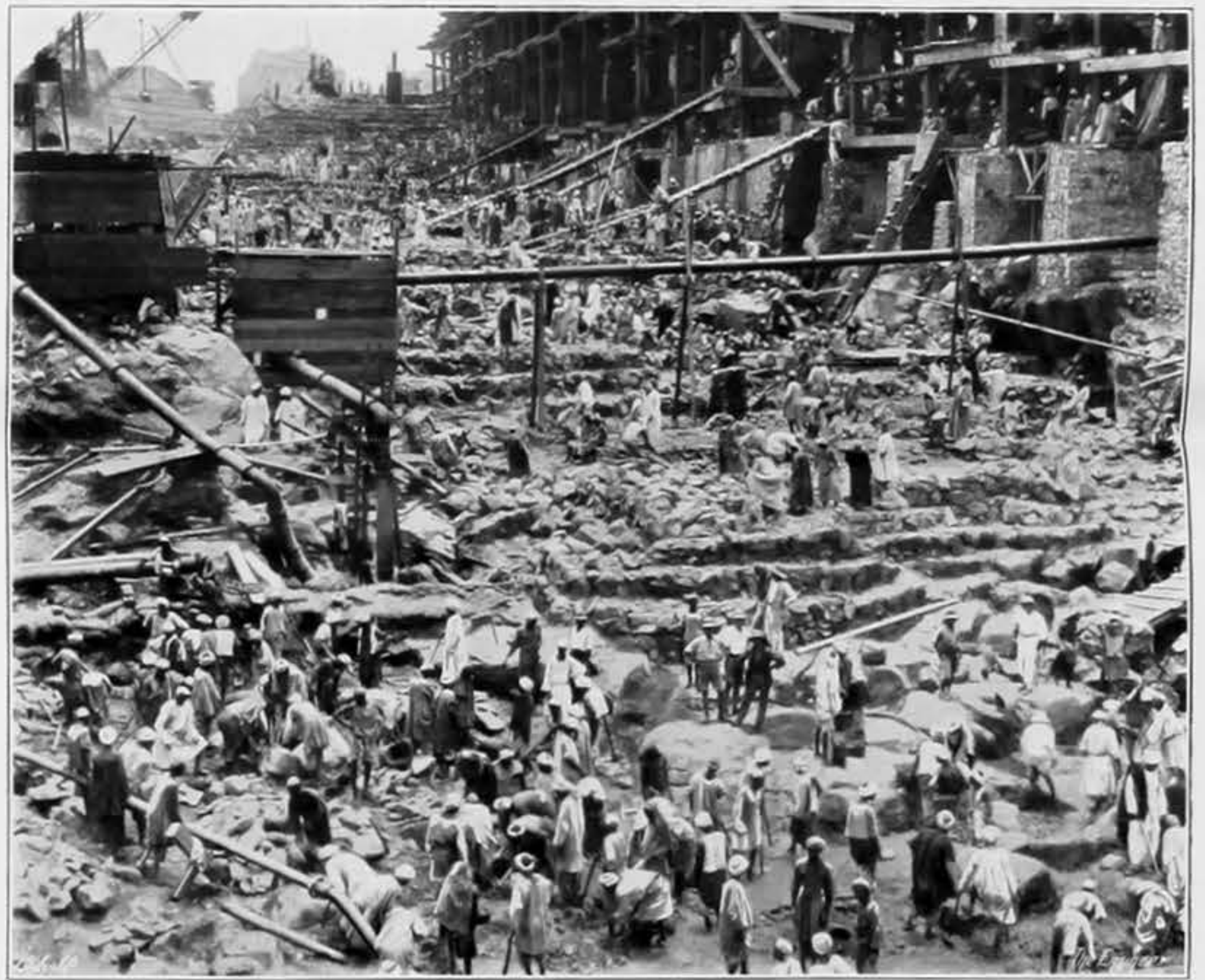
FIG. IV.—PROGRESS OF MASONRY ABOVE DEEP CHANNEL—APRIL 16, 1924
