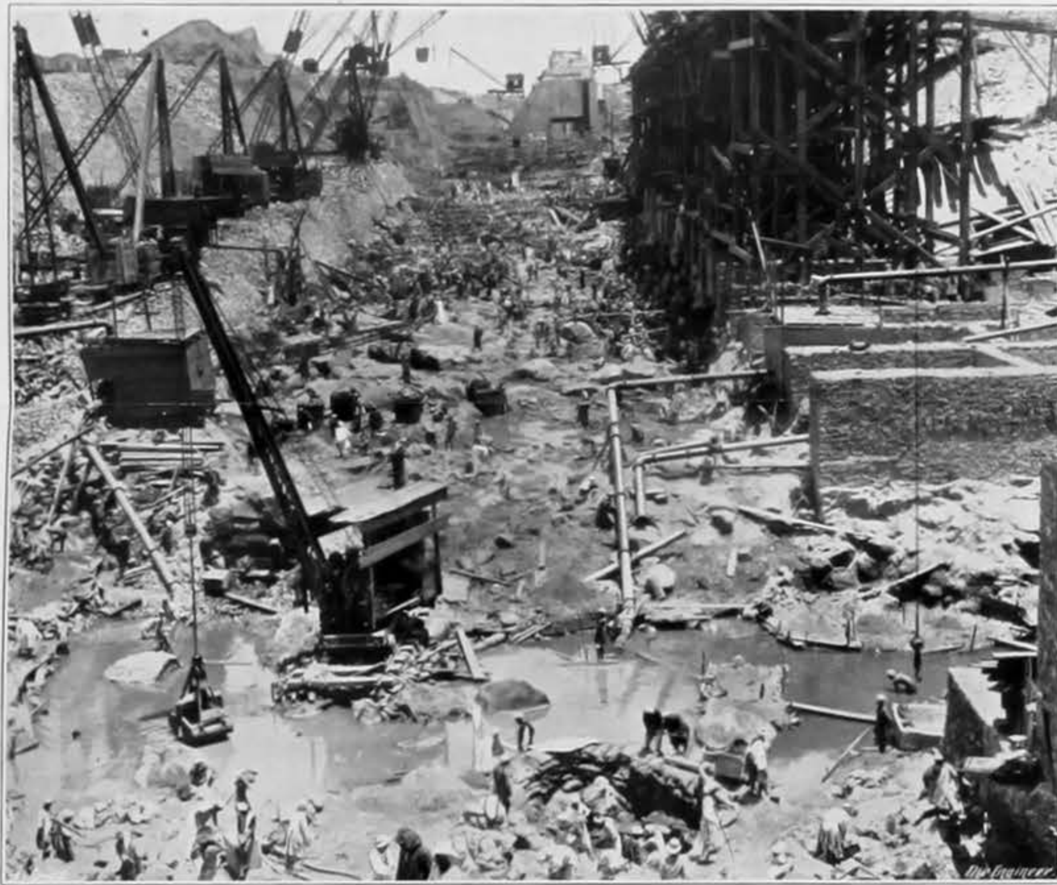
FIG. III.—LOOKING EASTWARD ACROSS PARTIALLY DE-WATERED DEEP CHANNEL—APRIL 1, 1924
