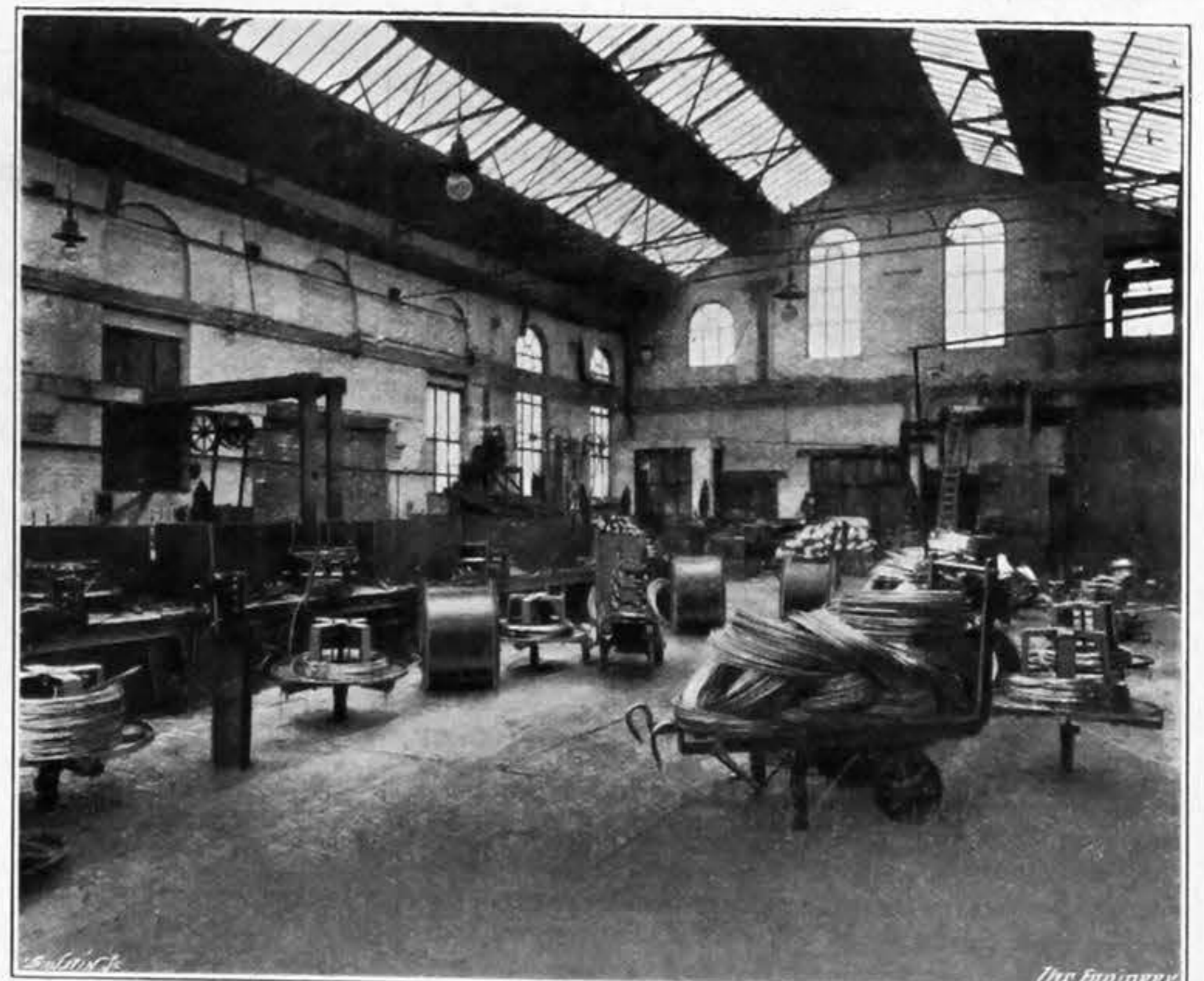
FIG. 78—HEAVY COPPER WIRE SHOP
