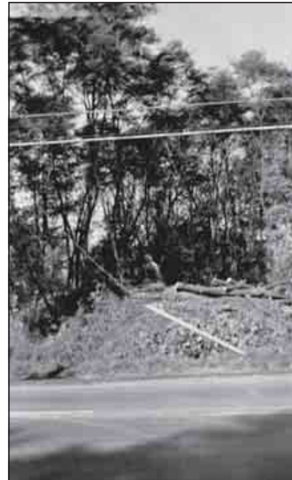
▲ Site of the Trenwill Building, 1950 (Phyllis Williams)
