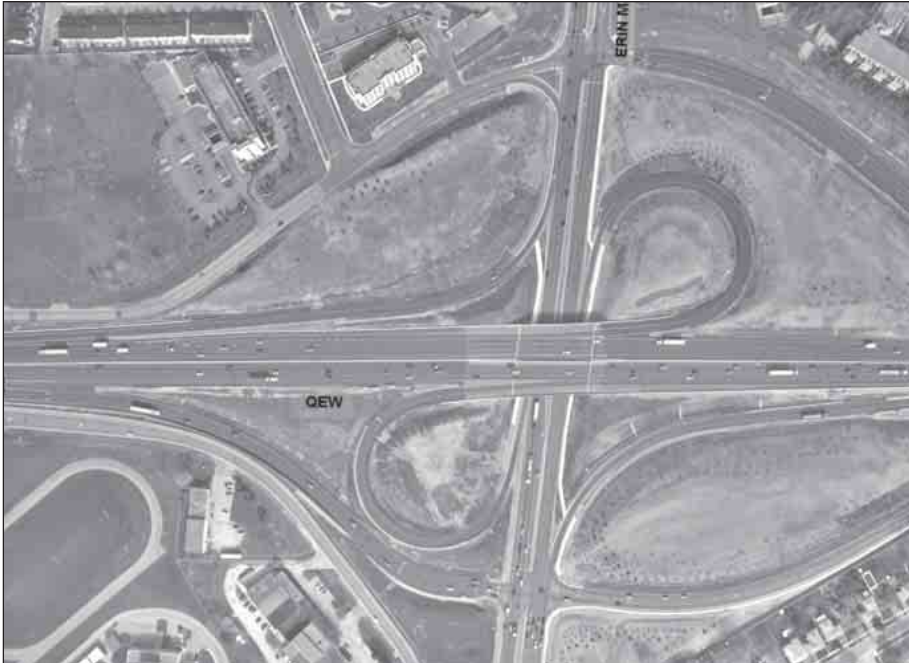
▲ Aerial View, 2002 (Ministry of Transportation)
