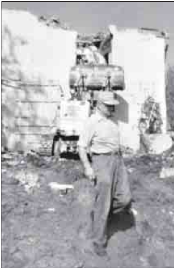
▲ Mr. Burton viewing demolition of Barrymede House
