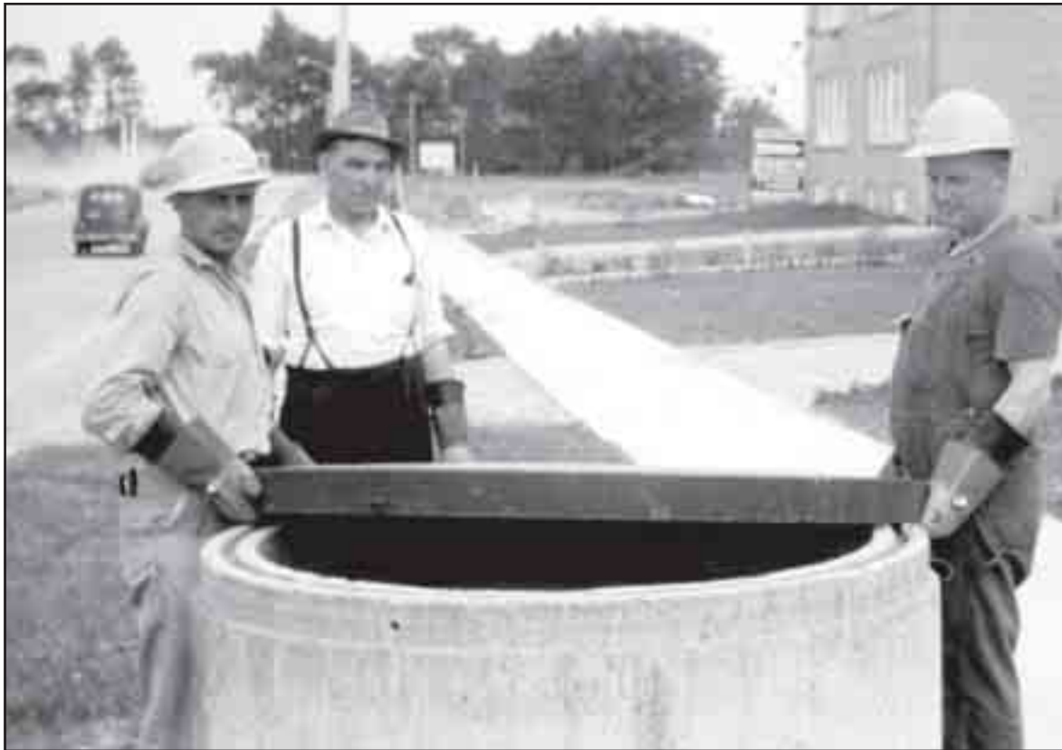
▼ Installing Hydro in Park Royal, 1957 (Enersource Hydro Mississauga)
