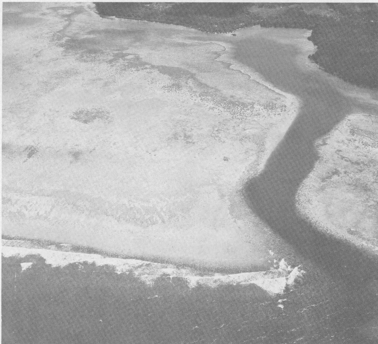
FIGURE 51.—Reef flat near Manell Channel. Most of this broad fringing reef off south Guam is covered by 1 to 3 feet of water during low tides. The seaward margin is rubby and does not contain well-developed algal grooves and spurs at this place. Photograph by U.S. Navy.
