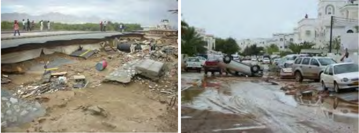
Fig. 4(a) Damage in Muscat in association with cyclone „GONU’
