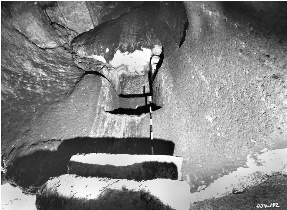
Fig. 3. The cistern opening closed by four stone slabs and the new entrance in the neck of the cistern closed with a stone slab (photo by S.J. Schweig, British Mandate record files no. 32)
