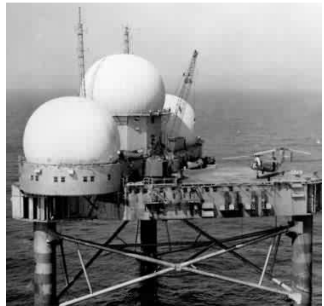
Fig. 4 – X-Bracing installed to stabilize TT4 (courtesy TTA)
