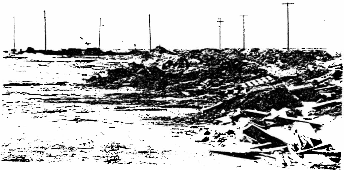
PLATE No. 7: View of miscellaneous fill and debris material on the study area adjacent to the present rail yards.
