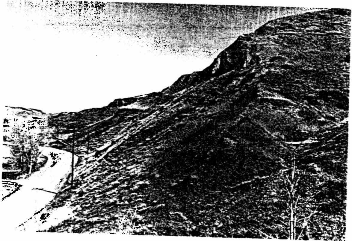
PLATE No. 3 View north of valley slope on the east side of the Oldman River showing typical slope profile.
