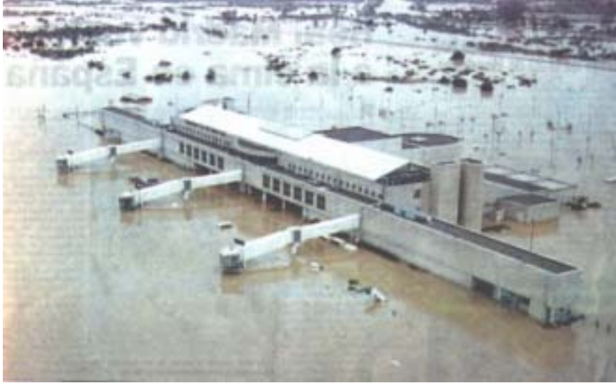
Photo 1. Airport in San Pedro Sula. Damage to facilities and suspension of services.
