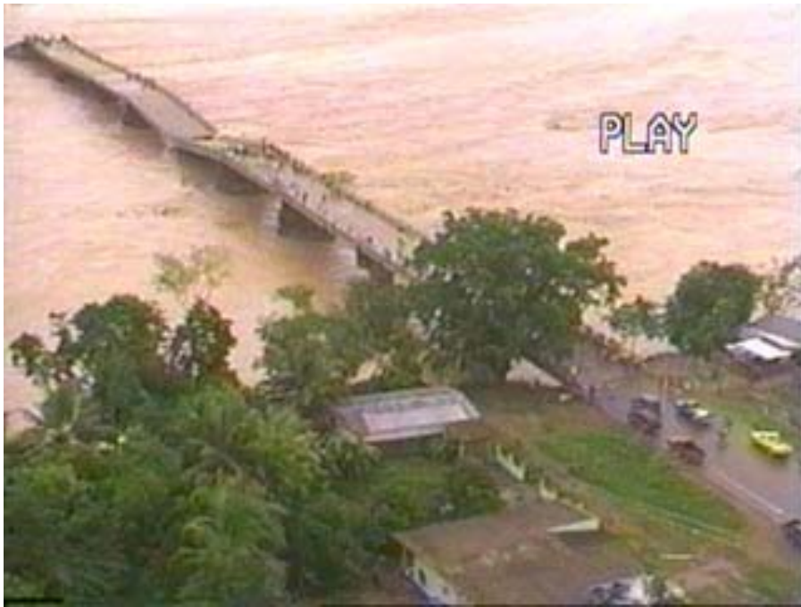
Photo 4. Destroyed bridge in the department of Colón.
