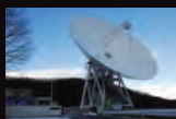
The 64-meter parabola antenna at Usuda Deep Space Center handled communications with Hayabusa.
