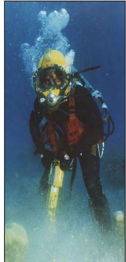
Figure 6-4. Underwater Construction Diving.
