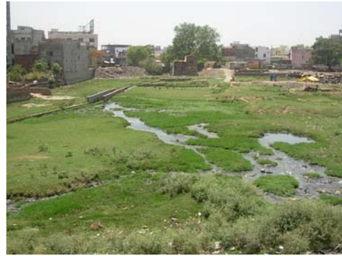
Leaking sewer line in the city
