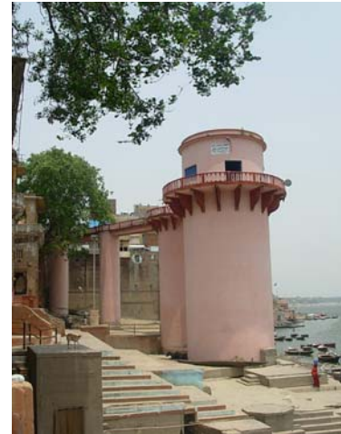
Intermittent Pumping Station at Ghat
