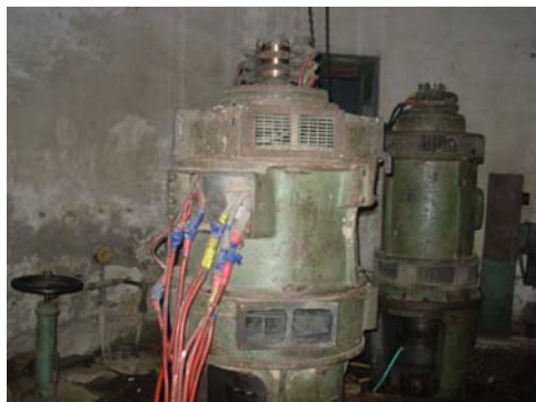
Deteriorated Conditions of Pumps
