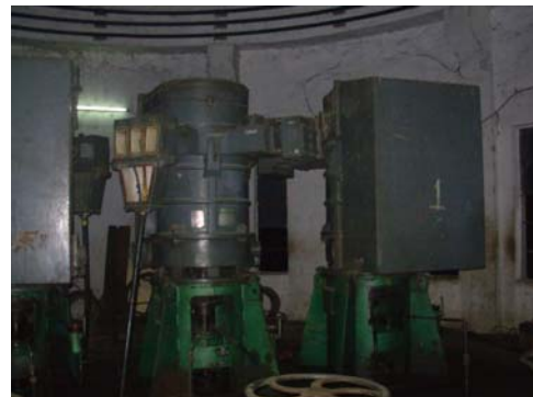
Deteriorated Conditions of Pumps
