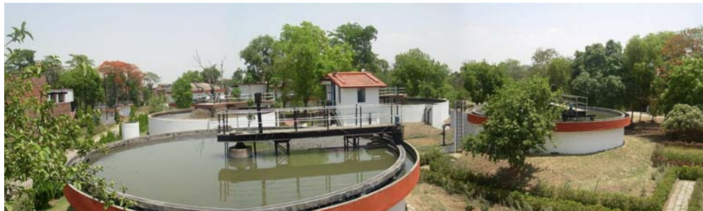
Sewage Treatment Plant at Bhagwanpur
