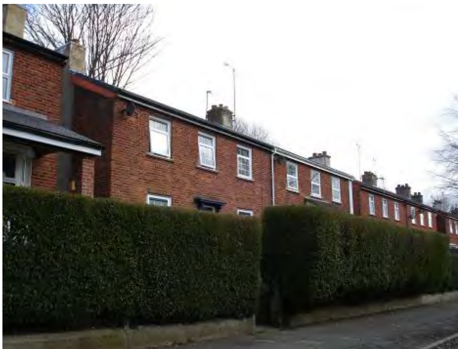
Figure 46: Steel framed council houses, Orchard Road
