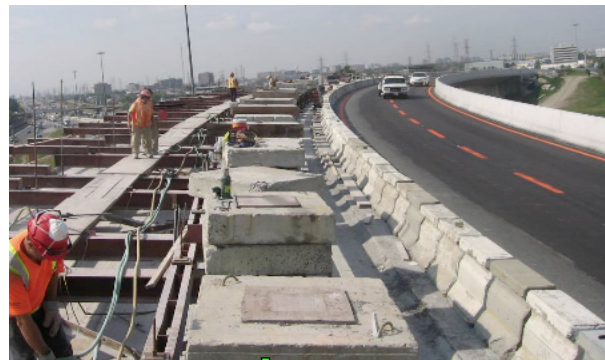
Construction of Highway 409
