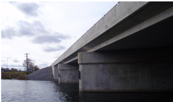
Scugog River Bridge
