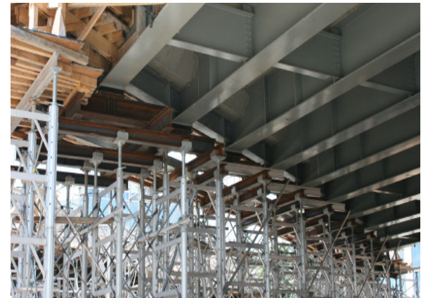
Carling Avenue Bridge preparation
