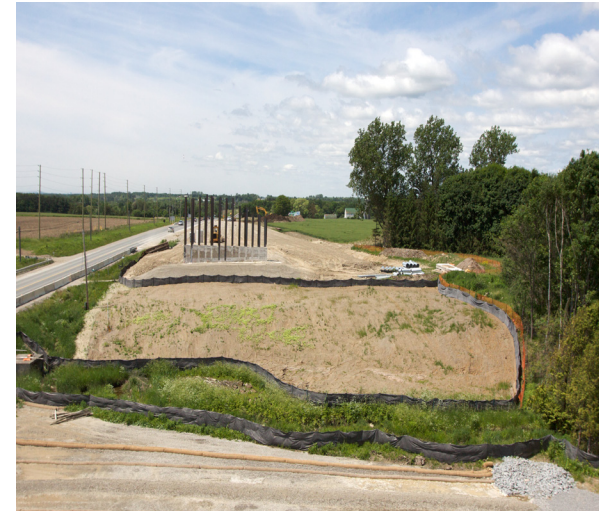
On-going work to implement Highway 407 East
