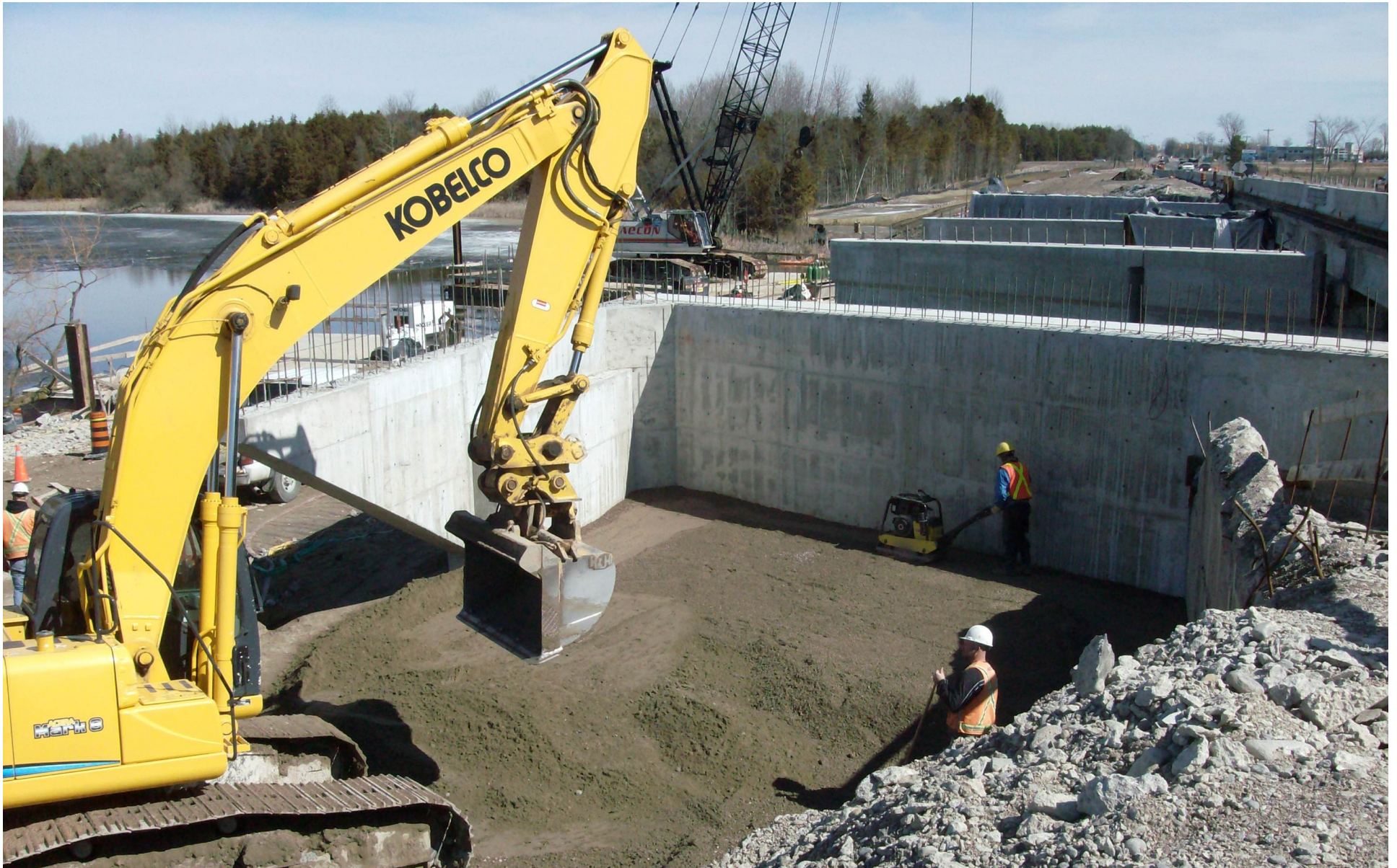
Highway 7, Scugog River Bridge, completed foundations
