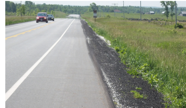
Highway 6, Paved Shoulders, Mar to Tobermory area
