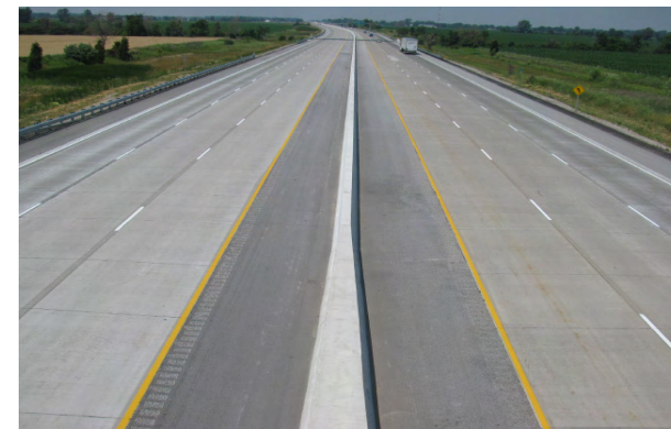
Hwy 401 widening and rehabilitation work completed
