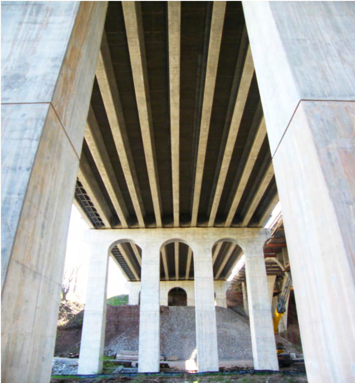
QEW Bridge Rehabilitation
