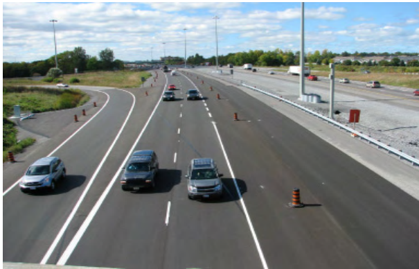
Hwy 417 widening underway
