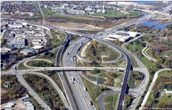
QEW to Red Hill Creek Expressway interchange completion
