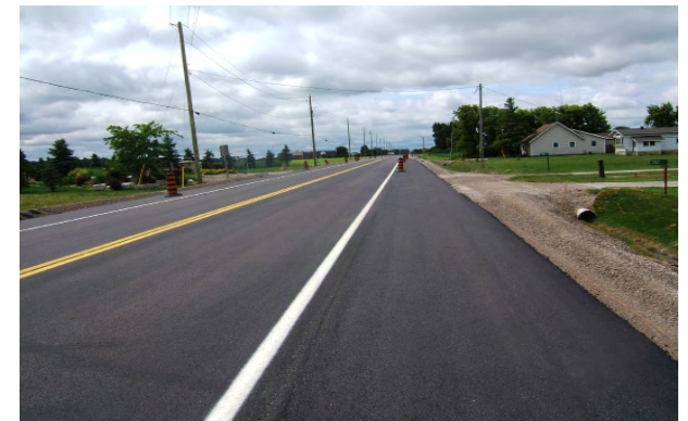
Hwy 77 rehabilitation improvements completed
