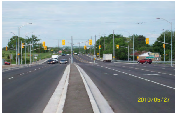
Hwy 7 completed improvements
