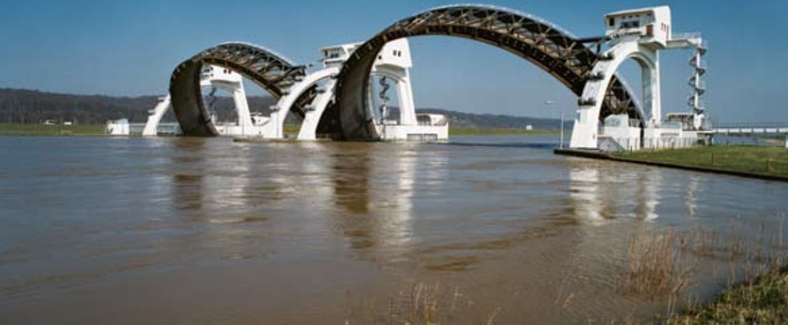
Weir in the Neder-Rijn at Driel.
