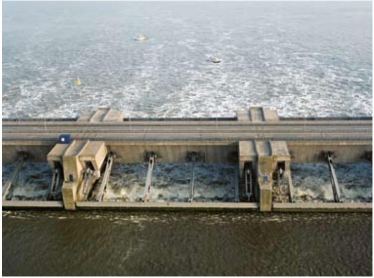
Sluice gates in the Haringvliet Dam. Together with the sluice complex in the Afsluitdijk and the one at IJmuiden, and with the weir at Driel, these sluice gates are key to the regulation of the discharge and distribution of freshwater.
