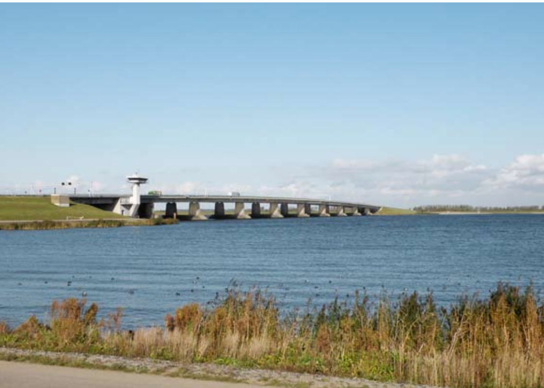
Bridge over Lake Ketelmeer.
