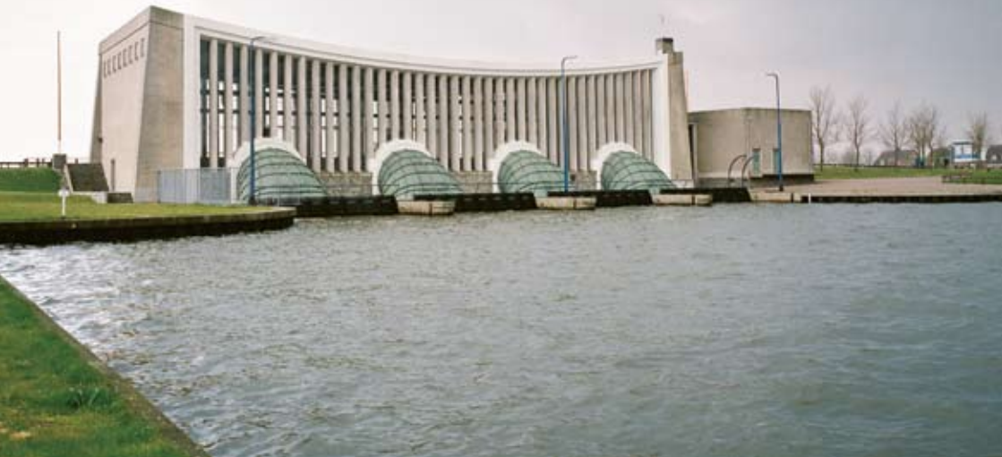
J.L. Hoogland pumping station at Stavoren. This is also an inlet point for the regional water system.
