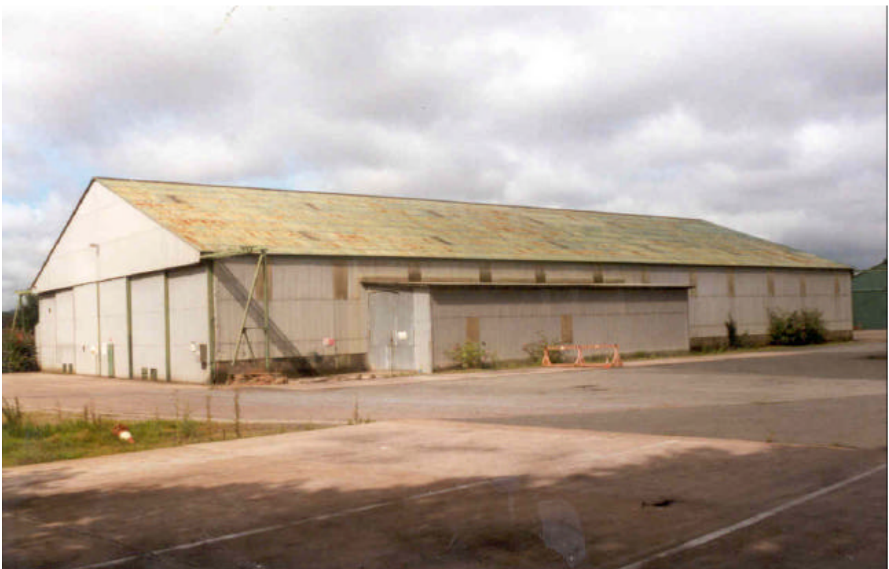
Photograph 2 - Type 'A1' Hangar
