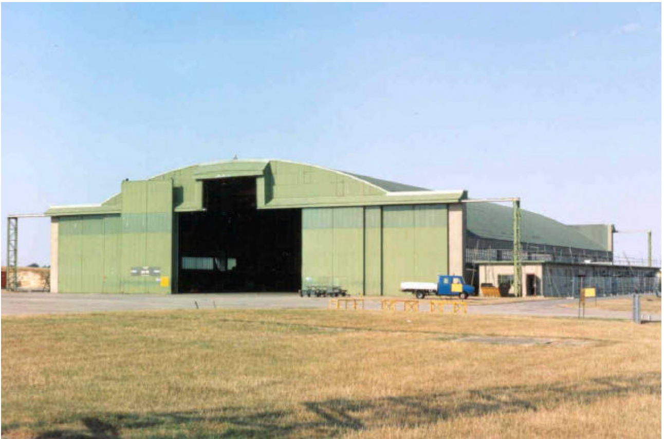
Photograph 13 - Type Gaydon Hangar
