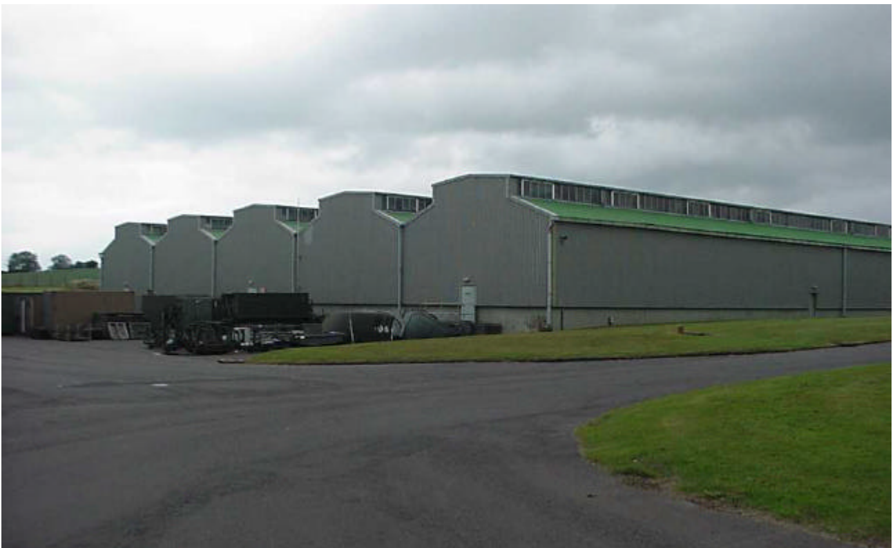
Photograph 22 - Type Quedgeley Hangar
