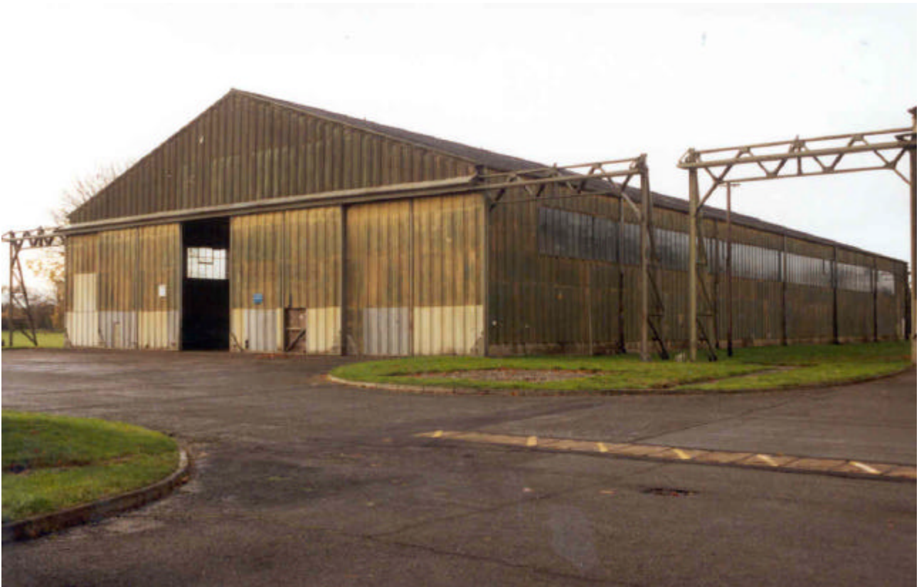
Photograph 14 - Type Hinaidi Hangar
