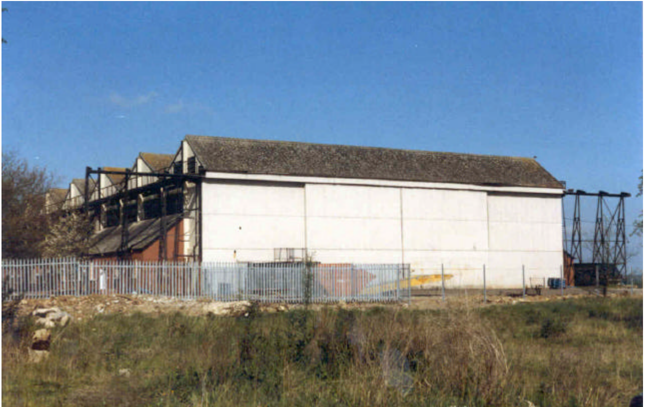
Photograph 1 - Type 'A' Hangar
