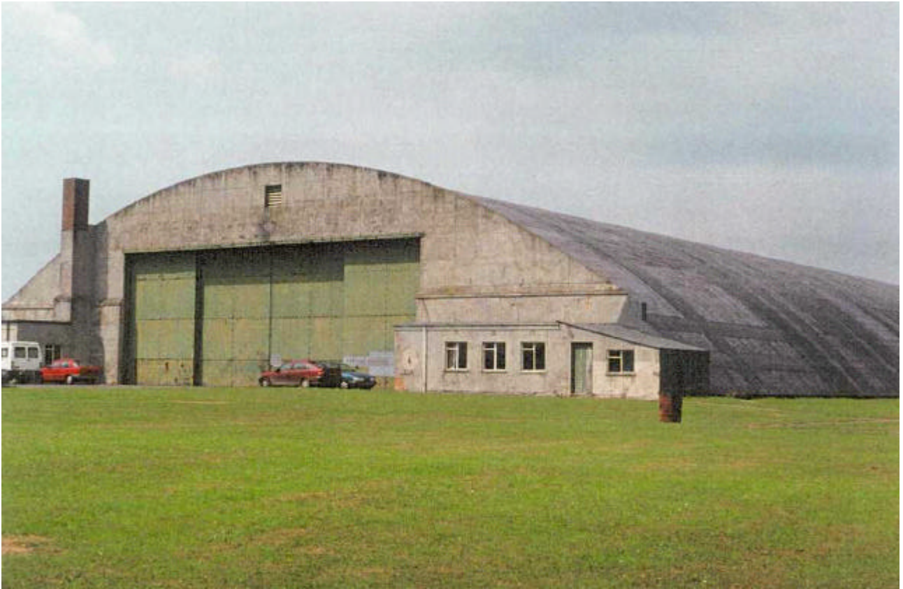
Photograph 17 - Type 'L' Hangar
