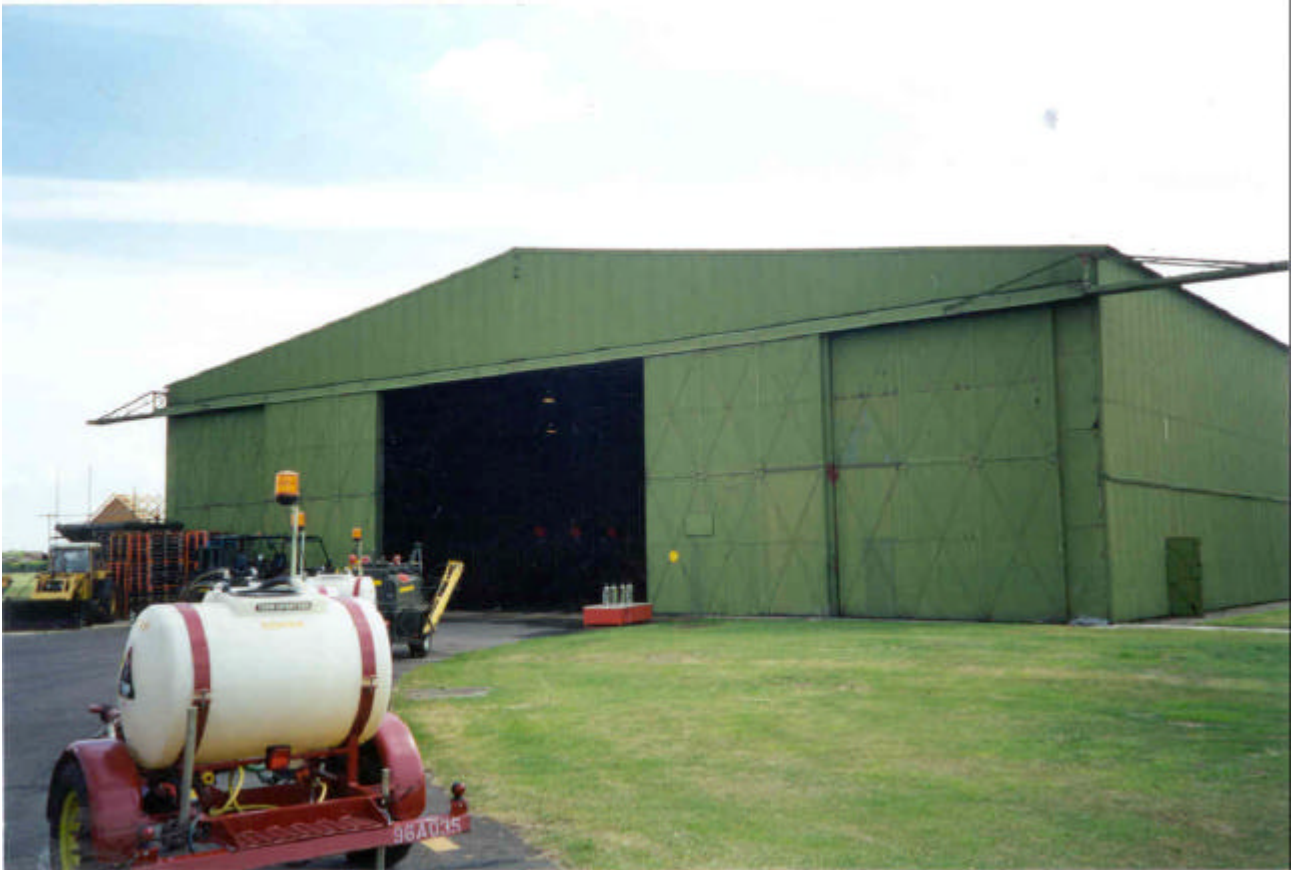
Photograph 23 - Type T2 Hangar
