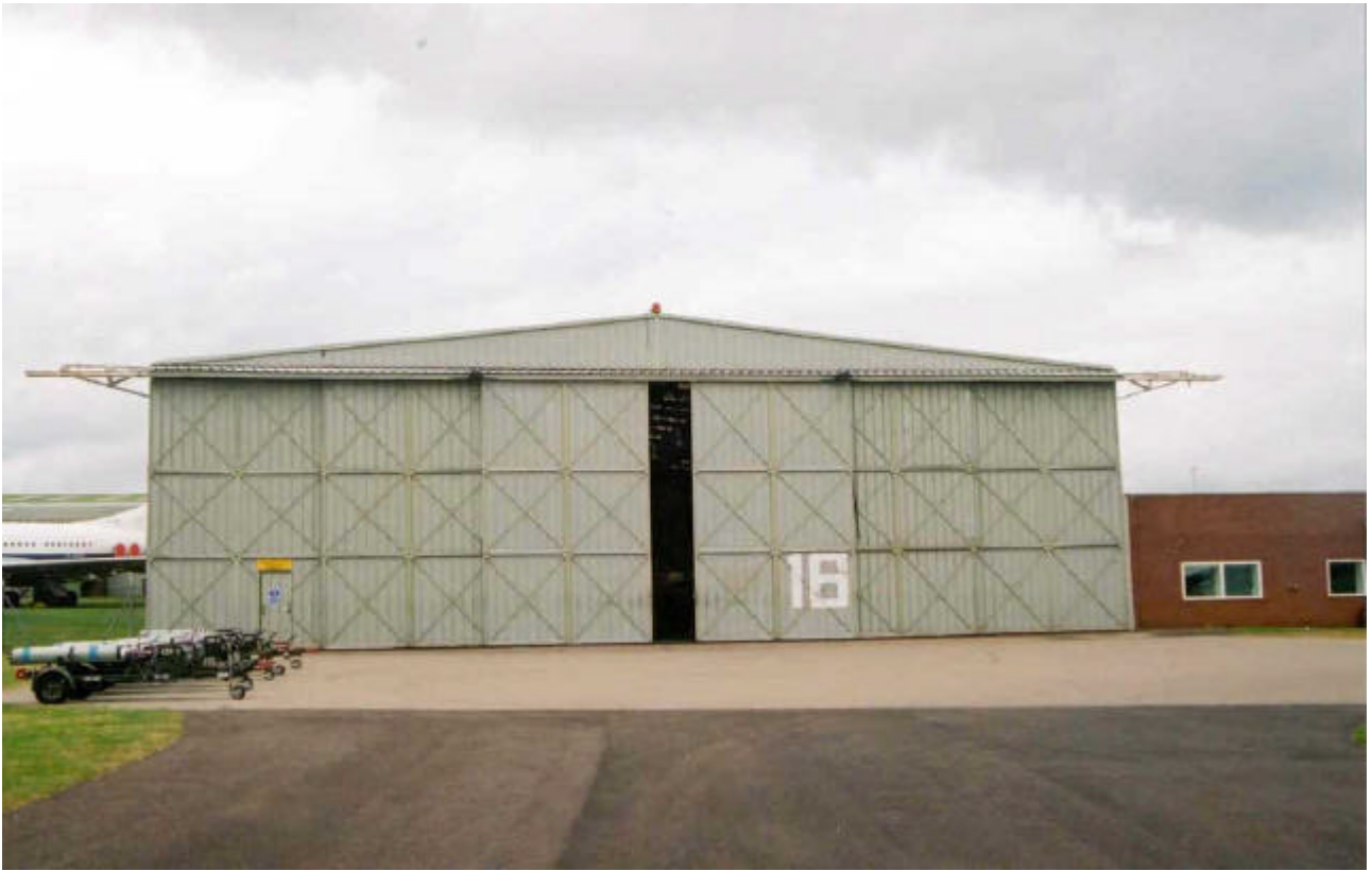
Photograph 5 - Type Bellman Hangar
