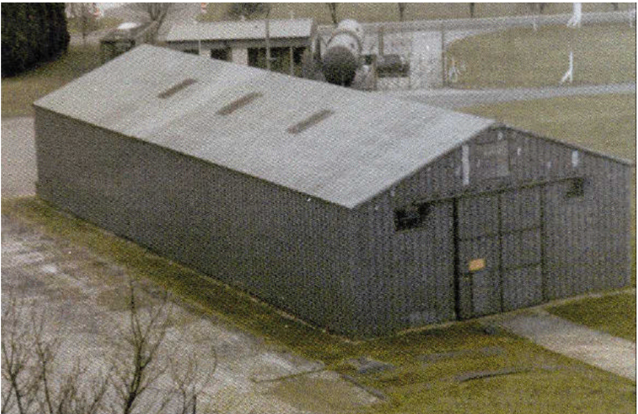
Photograph 6 - Type Butler Shed
