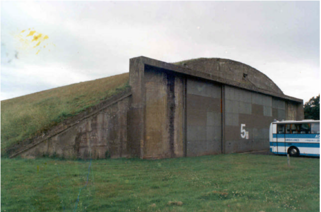
Photograph 11 - Type 'E' Hangar
