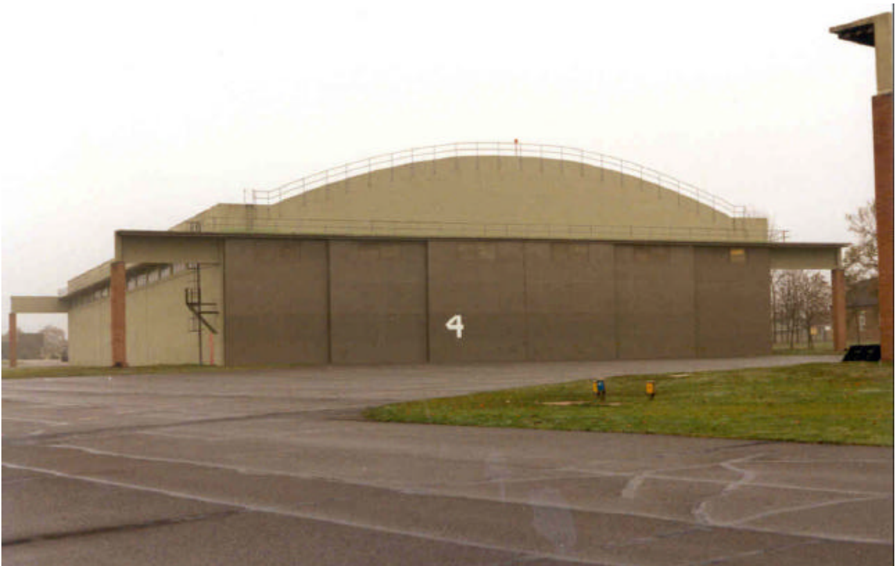
Photograph 10 - Type 'D' Hangar
