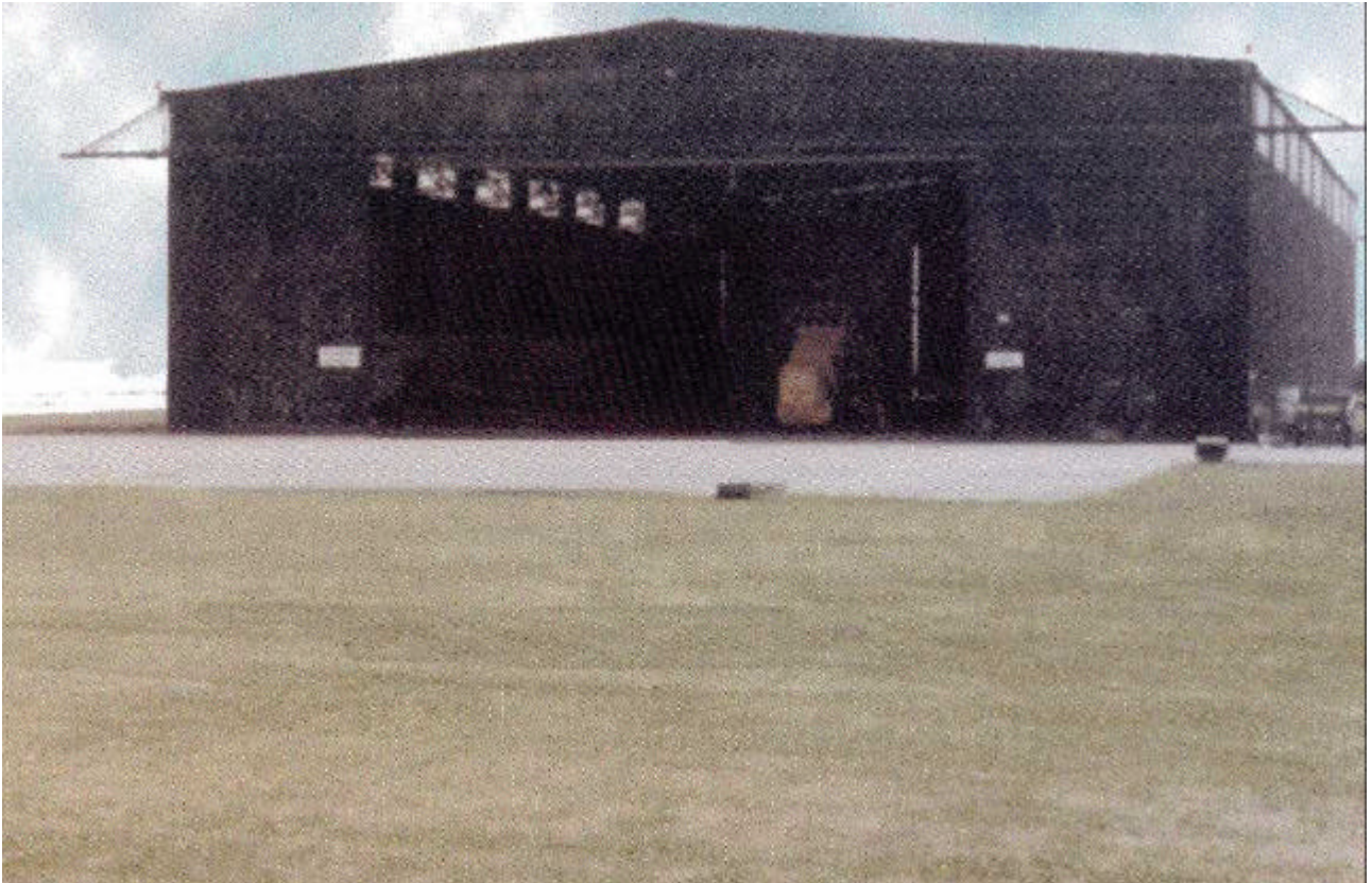
Photograph 9 - Type Callender Hamilton Hangar
