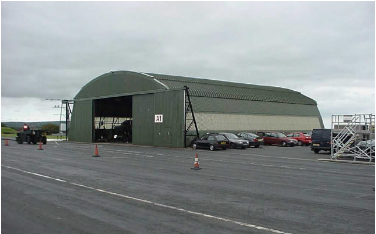
Photograph 19 - Type Mainhill Hangar
