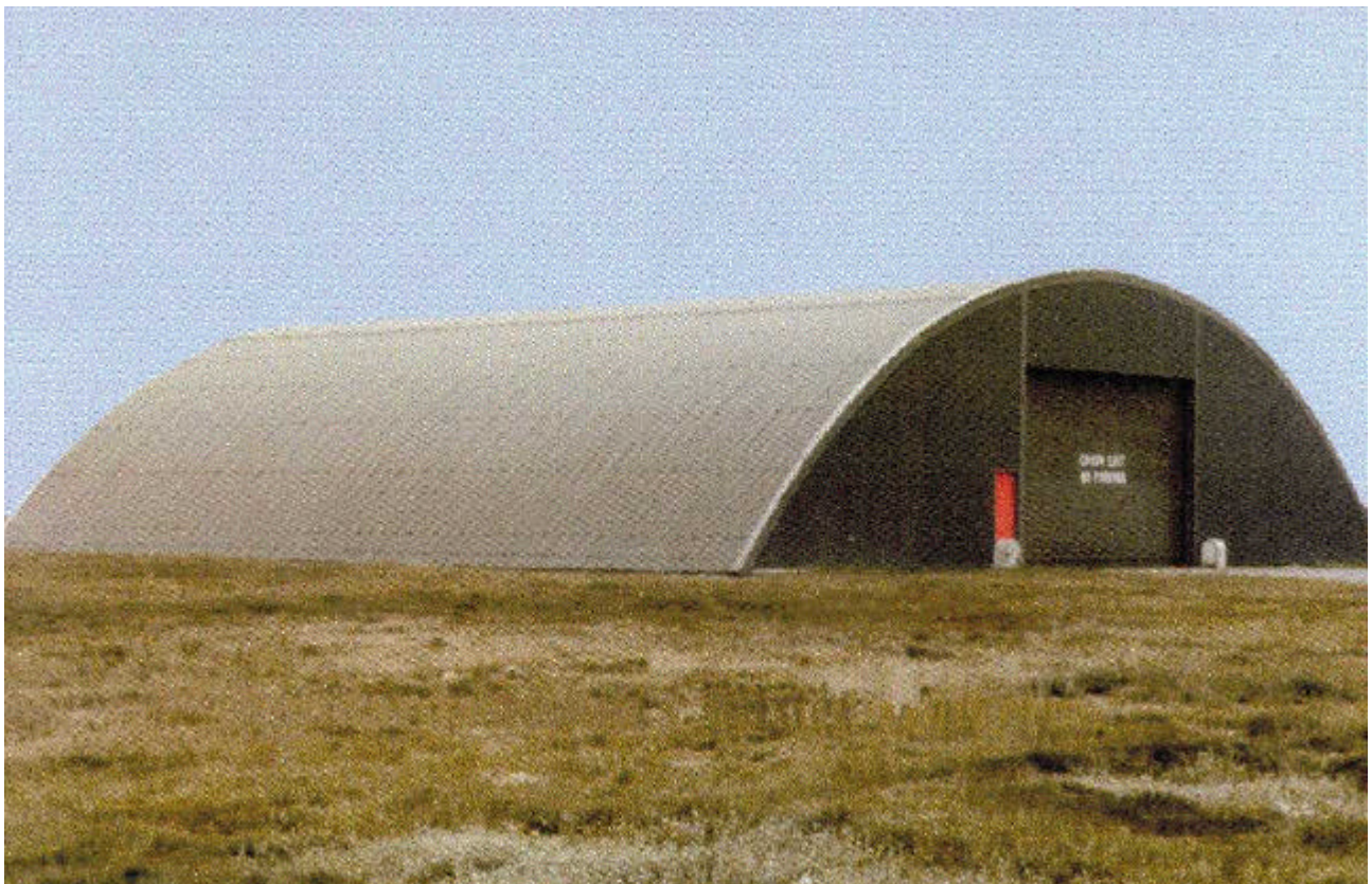
Photograph 20 - Type Miskin's Blister Hangar
