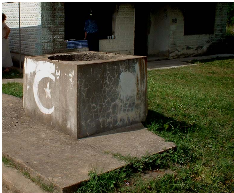
Fig. 5. Farm well in Bukvik, Brčko District June 2003.
