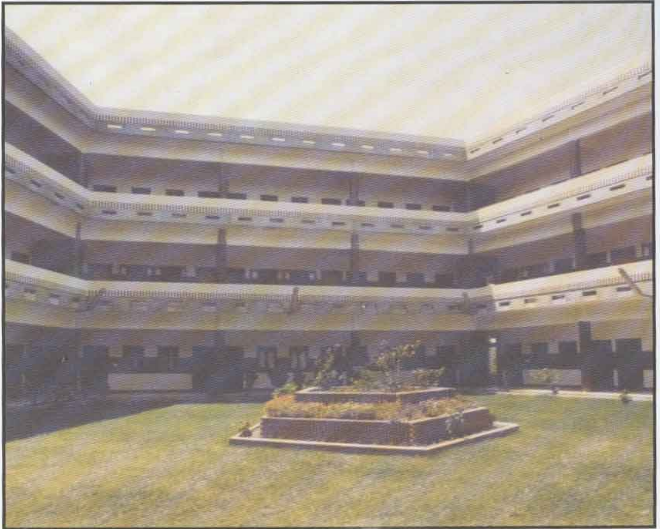
Interior View of the Impressive three Storied of New Classrooms
