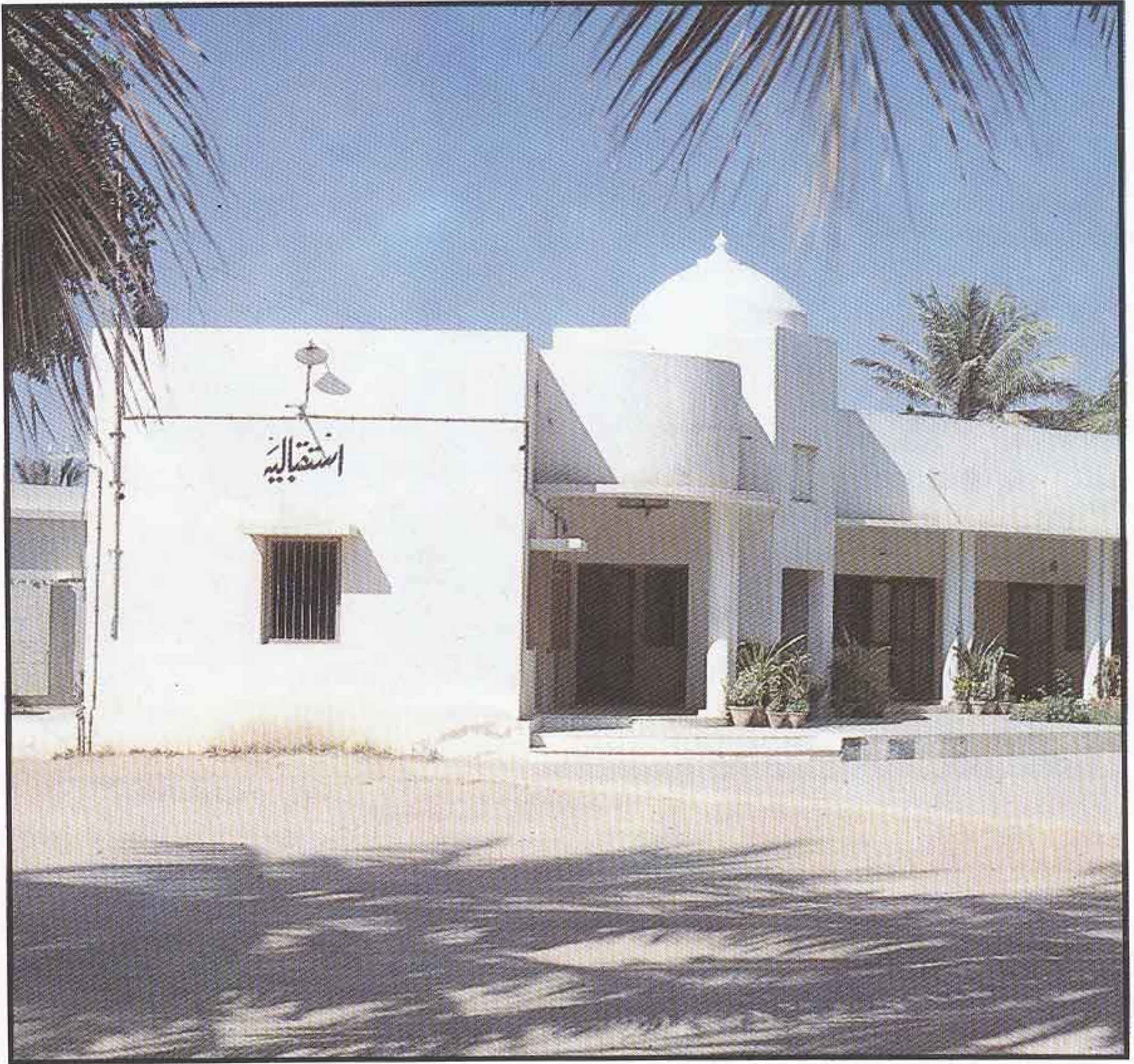
Reception, Telephone Switchboard and other Managerial Offices
