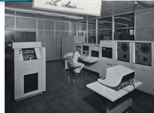
One of Eurinfor's computer rooms
