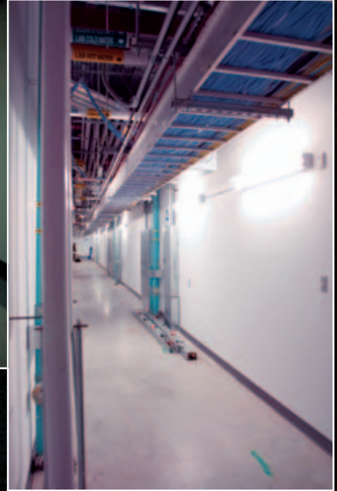
Hallways behind labs permit rapid change of utility and data service.
