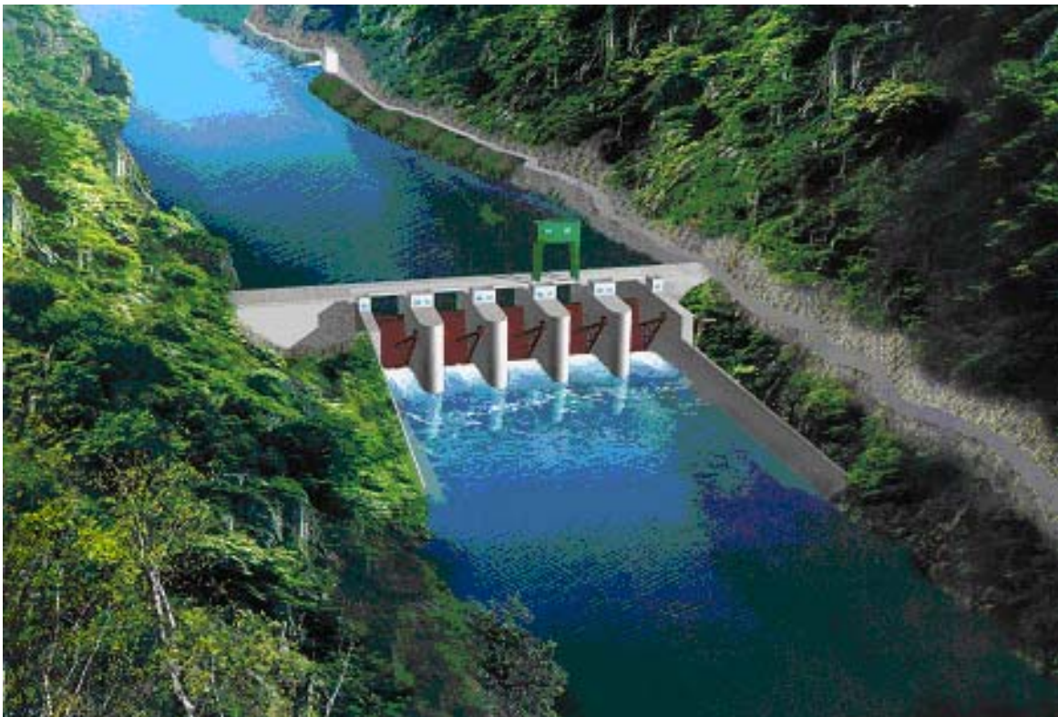
Bird's view of Jinping-II Project
