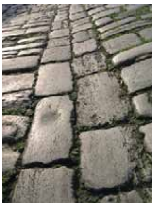
Purbeck paving, Kings Bench Walk
