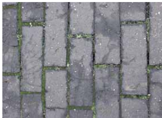
Wood Paving at Chequer Street EC1
