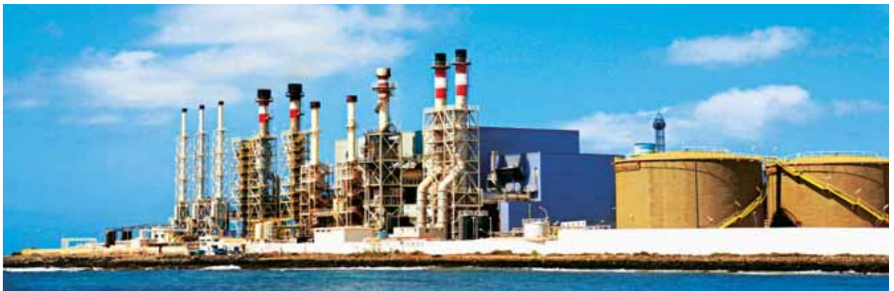
Thermal desalination plants are part of L&T's capabilities in the water sector
