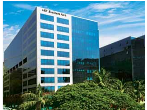
L&T Business Park at Powai, Mumbai
