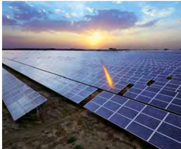
Solar Photo Volatic (PV) power Plant commissioned by L&T
