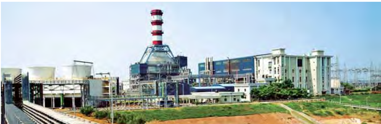
Natural gas-fired combined cycle power plant built by L&T at Vemagiri in Andhra Pradesh, India
