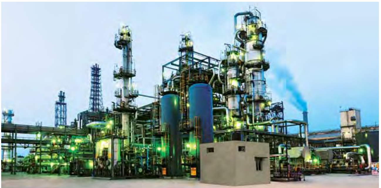
900 tpd ammonia plant of National Fertilizers Limited, Panipat - one of the many downstream hydrocarbon projects executed by L&T, on a licence plus EPC basis
