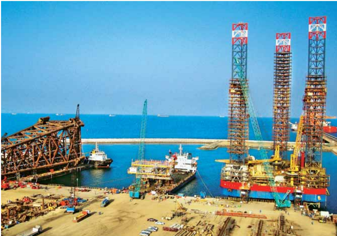
L&T's modular fabrication facility at Sohar in Oman has the capability to execute large scale fabrication up to 20,000 tonnes. Picture shows a jacket, a platform and a jack up rig.
