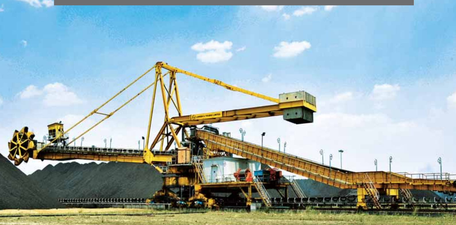
Coal handling plant executed by L&T at Koderma in Jharkhand. L&T is a single point solution provider for a comprehensive range of material handling systems.
