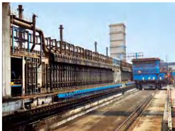
Coke Oven Battery at one of India's major steel plants.
