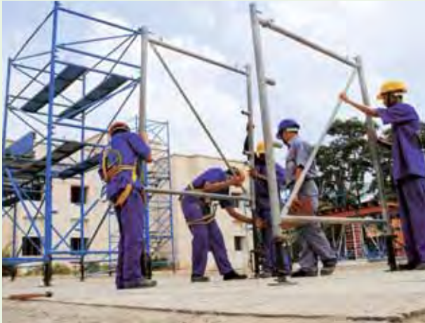
Scaffolding erection training at CSTI, Chennai
