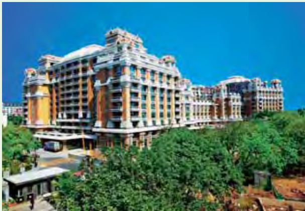
L&T has constructed ITC's 600-room five-star hotel - the world's largest LEED-certified green hotel
