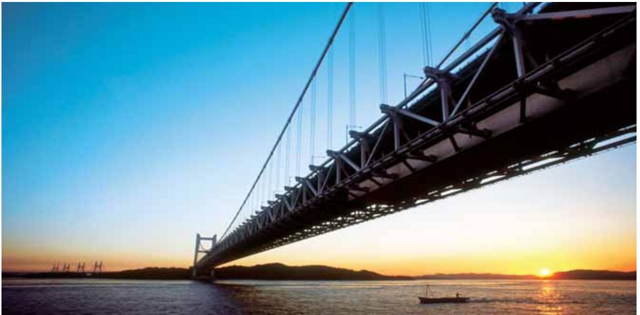
L&T's capabilities in bridge-building include design and construction of many types of bridges of different span lengths using innovative techniques and construction methods.
