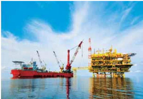
L&T's heavy-lift-cum-pipelay vessel LTS 3000 installing a topside for Newfield Peninsula in Malaysia.
